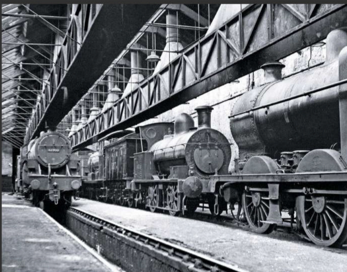
An LMS 'Crab' and '4F' flank an LNER 'J17' and LNWR Ramsbottom O-4-OT within Hellifield shed in 1965, while the rear of 'V2' Green Arrow's tender is also just visible. The remote location made this an ideal storage facility for locomotives destined for the National Collection. RAIL PHOTOPRINTS
