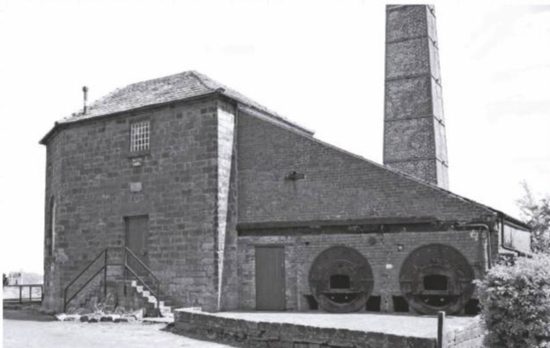
Below: The engine house was built in 1829 by the Butterley Company to haul wagons up Middleton Incline and is constructed from dressed Gritstone blocks with a pitched slate roof. The adjacent boiler room has a single pitched roof made of tiles with walls from blue and red brick. Much greater detail and approximate footprint sizing is available at https://her.derbyshire.gov.uk/MONUMENT/MDR9457
