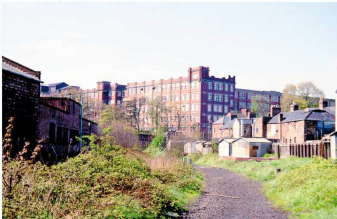
Above: Rowntree's factory, as it faces onto the branch line, was referred to as the Almond Block and extension, dating from 1911. It was a large reinforced concrete-framed building, clad with smooth red brick in English Garden Wall Bond and ashlar York stone for decorative features. The left-hand section seen here has been demolished.
