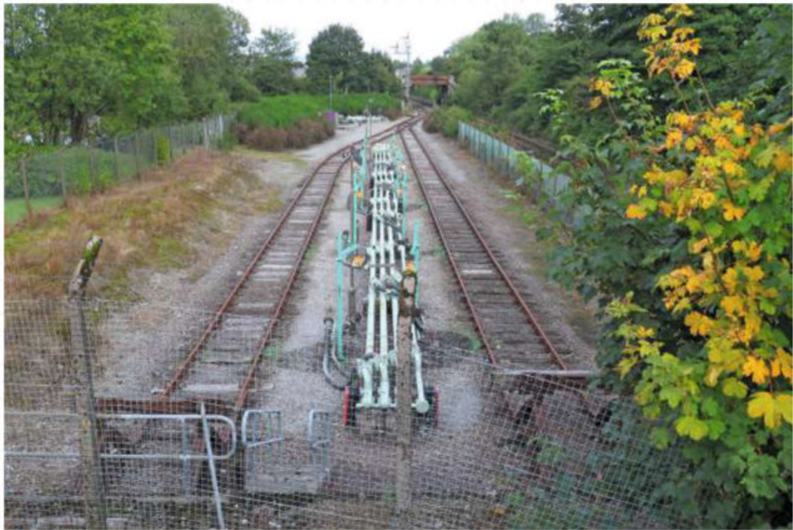
Below: Fort William oil terminal looking towards Fort William junction. Due to the sensitive and volatile nature of oil, the entire site is protected by a security fence.
