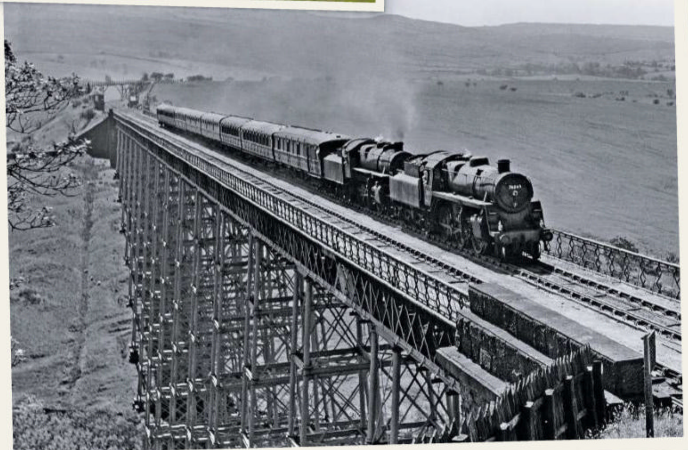
One of the Stainmore Route's most famous structures was the iron viaduct over the River Belah, which was designed by infamous bridge engineer Thomas Bouch of Tay Bridge disaster fame. Standard '4MT' No. 76045 leads an Ivatt classmate over the structure - which is now but a memory - with a holiday special returning from Blackpool to the North East in the 1950s. CECIL ORD/RAIL ARCHIVE STEPHENSON
