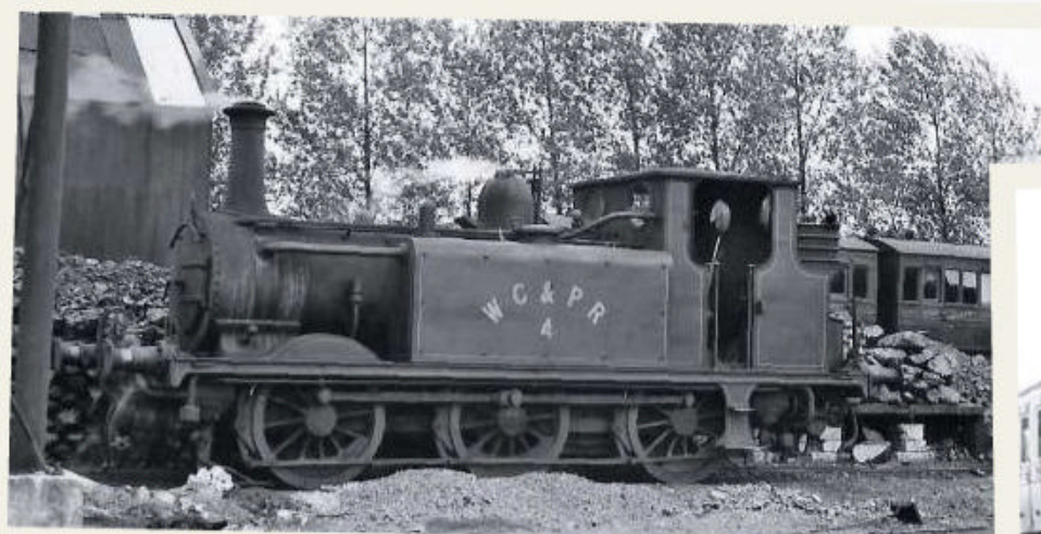
Above: Clevedon station was the railway's nerve centre, with locomotive and carriage sheds and, just a few hundred yards further on, a siding to the town's gas works. WCPR No. 4 stands outside the shed on June 25 1938. One of the tracks in the foreground curved round behind the shed to reach the GWR's Clevedon station. CHRIS LEIGH COLLECTION
