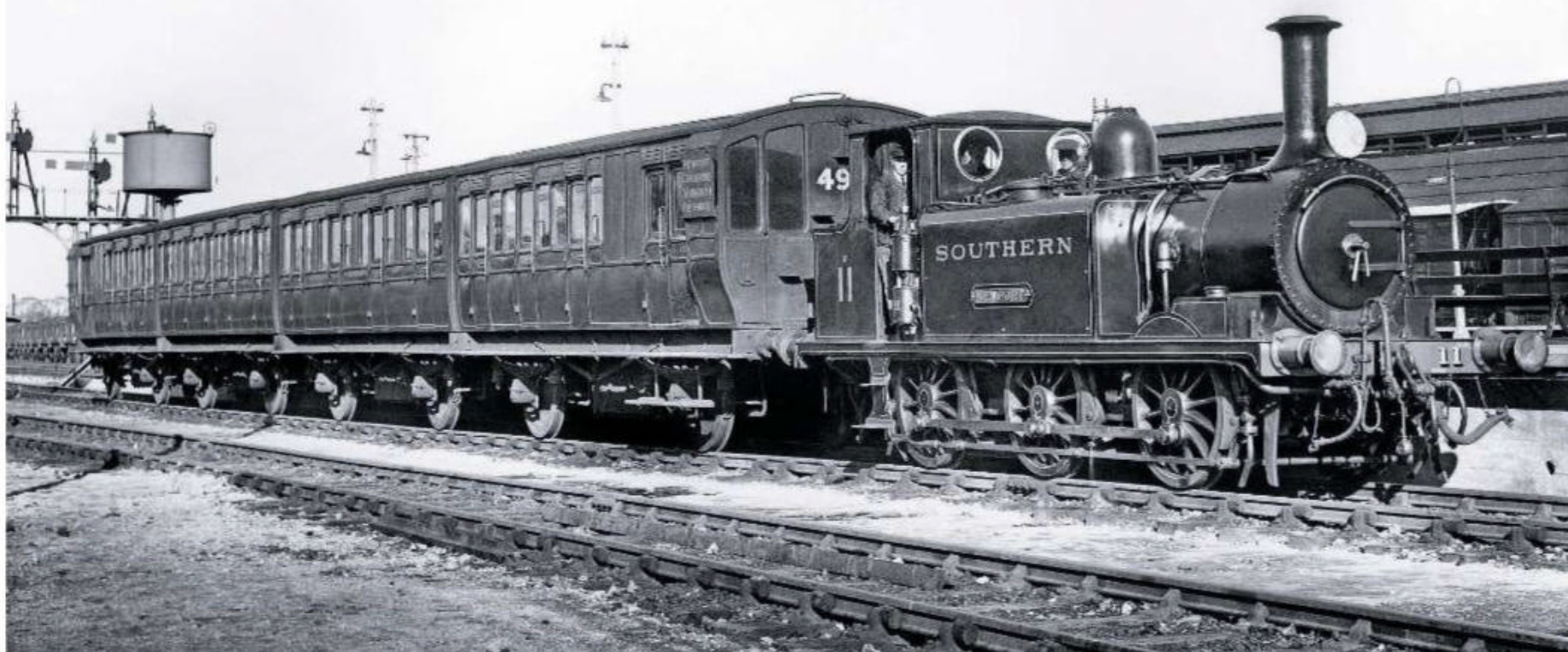
O.J. MORRIS/RAIL ARCHIVE/STEPHENSON
