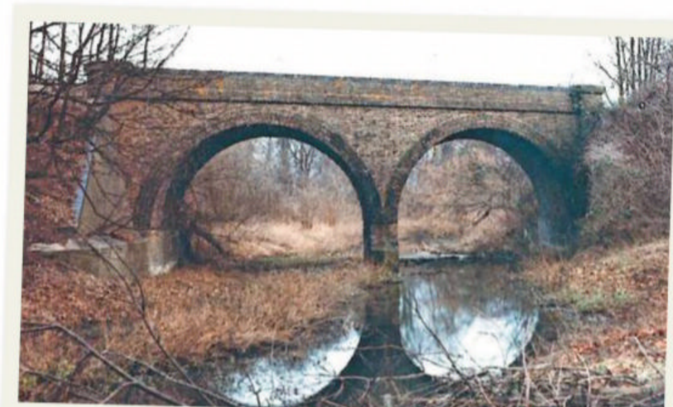
The Wyrardisbury river bridge shortly before its demolition in 1981. Periodic clearances of the channel were needed, particularly through the left-hand arch. CJL COLLECTION
