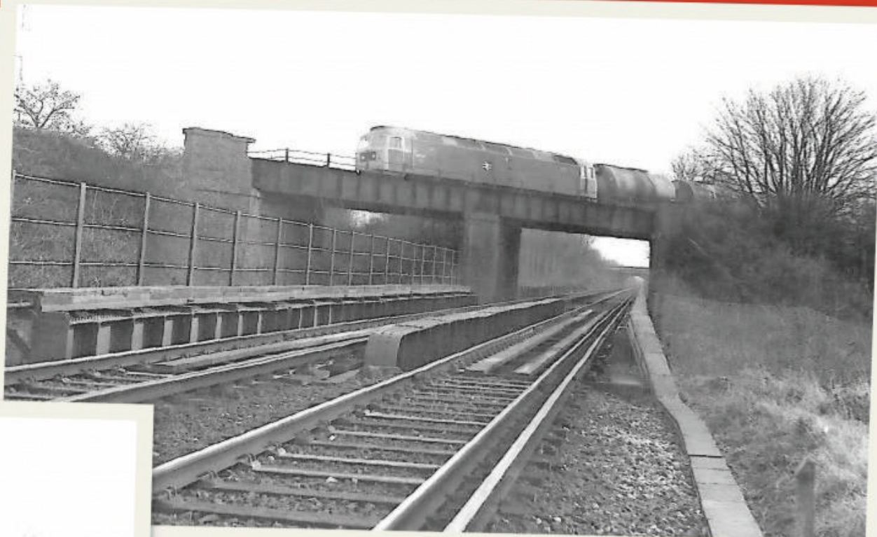
Above: This view from a public foot crossing that has since been closed, shows that, though the girders are a single, full-width span, there is a supporting brick pier in the centre. CHRIS LEIGH
