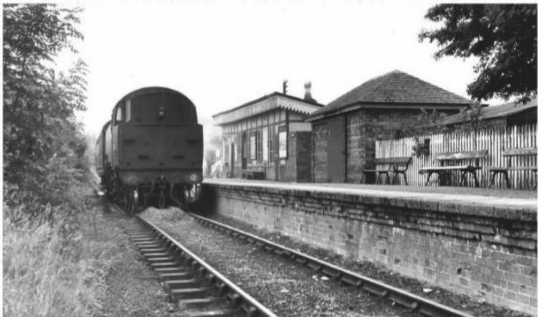
Below: Killin station itself was rather delightful. This is the view looking towards Killin Junction. Behind the photographer is the line to Loch Tay, where the locomotive was stabled and serviced. '4MT' No. 80093 will move into the yard behind the photographer to allow the coach to roll past; it will be collected by No. 80093 for the journey to Killin Junction. JOHN GOSS
