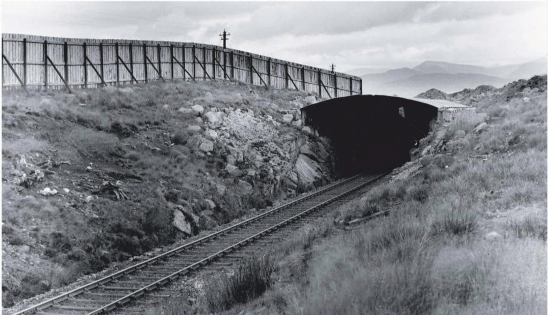
Below: Britain's only railway snow shelter is at Cruach Rock, near Rannoch, on the West Highland Railway, pictured in this photograph taken in or around the 1930s. Note the snow 'fence' to the left, which was aimed at combating driving snow. GETTY
