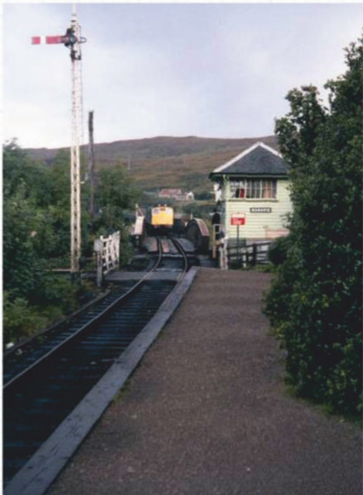
Above: Banavie swing bridge over the Caledonian Canal, and its neighbouring station, sit in the shadow of Ben Nevis. It's of bow string construction and was originally turned by hand (but is now hydraulic). An unidentified Class 25 on passenger duty reduces down to the mandatory 5mph speed restriction over the bridge on September 26 1979. PAUL A. LUNN COLLECTION
