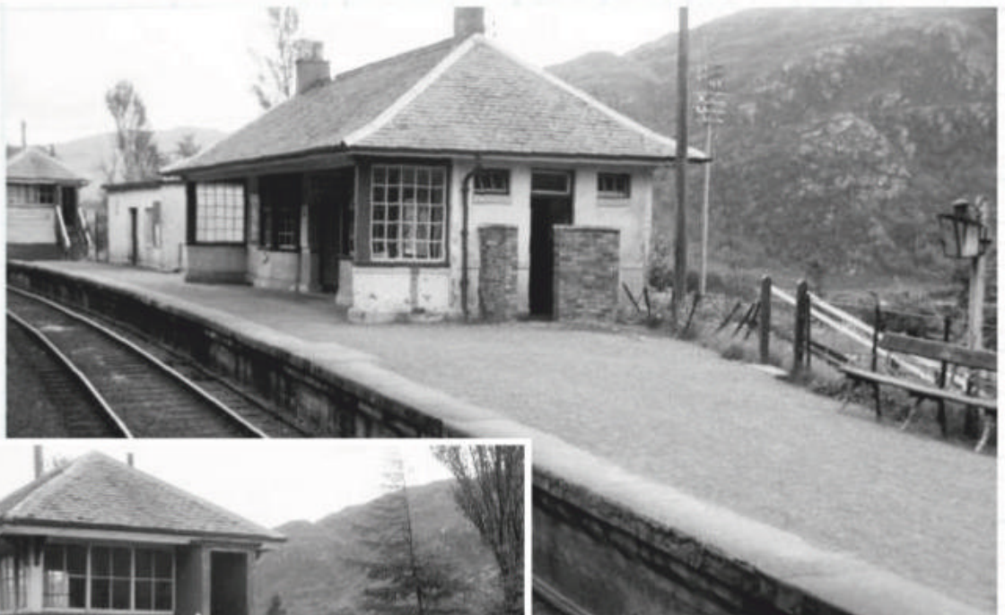
Above: Glenfinnian station has two platforms, linked by a foot crossing, a passing loop, headshunt and two sidings. PAUL A. LUNN COLLECTION
