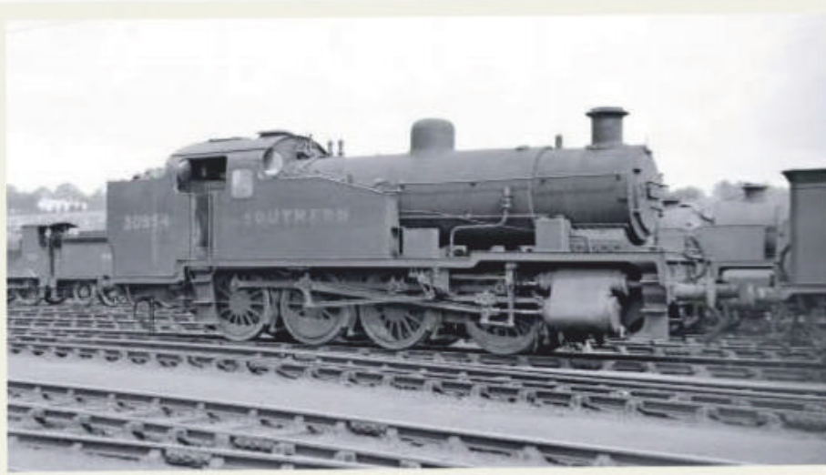
Left: No. 951 sports smart Southern Railway wartime black outside Eastleigh Works circa 1946/1947. The protrusion behind the chimney is a valve designed to allow any condensed steam to escape, a job normally performed by the cylinder draincocks. However, this valve lifted such steam clear to improve visibility from the cab. Fitting started in 1939 but they were removed from 1946. RAIL ARCHIVE STEPHENSON
