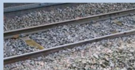
While we generally aim to have very little ballast chippings on top of the sleepers, sometimes even the real railway doesn't get it quite right!
