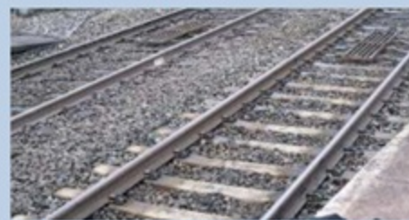
Real ballast on the West Coast Main Line. Although predominantly grey, the weather and passing trains have affected the shade.
