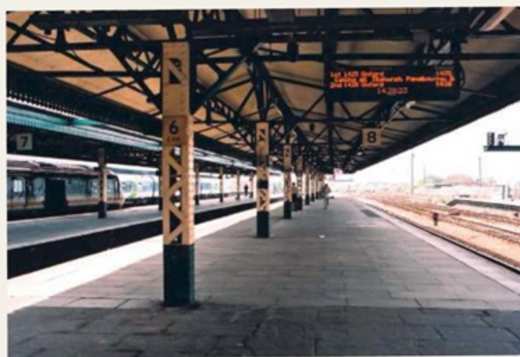
Above: The canopy at Reading General has been cut through to provide clearance for a new footbridge, which gives a clear view of the shape and construction of the structure. CHRIS LEIGH
