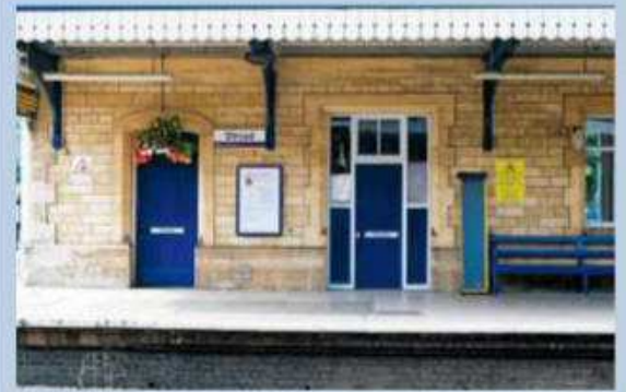
Stroud's platforms comprise modern paving slabs with engineer's blue brick 'walls'. CONVERY FLOWERS/ALAMY
