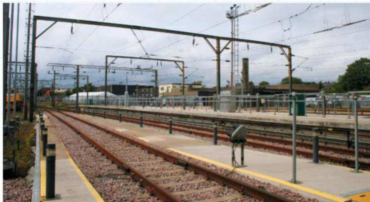
Left: Immaculate track at the north end of Willesden depot. All depots are provided with concrete walkways, and overhead catenary is a must.
