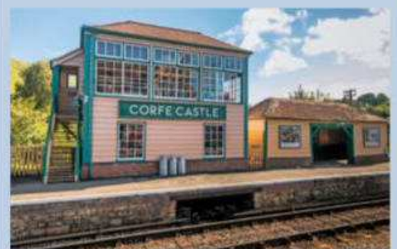
Corfe Castle's platform 'walls' are made from dressed stone, topped by layers of brick. There's also minimal overhang of the coping stones. STUART C. CLARKE/ALAMY
