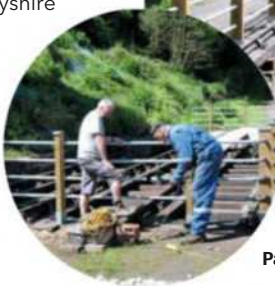
Inset: Blacksmiths Ian and Mark Baxter build a new fence to protect the pit at High Peak Junction, the pit which holds the remaining winding wheels and adjusters for Sheep Pasture Incline. PAUL A. LUNN
