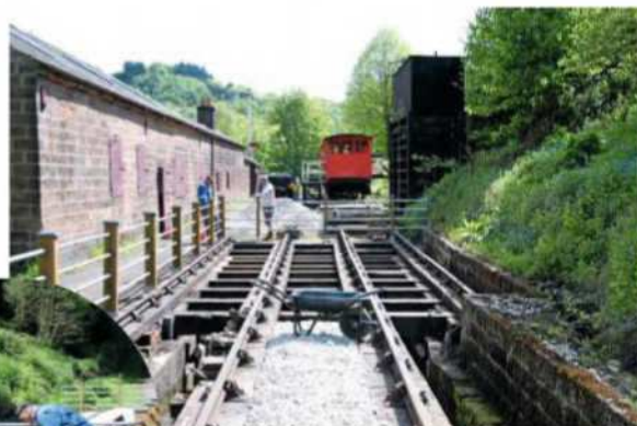
Above: The restored pit at High Peak Junction. The workshop buildings are on the left. The wall on the right was a post-closure repair that inadvertently severed what remains of the ascending track up Sheep Pasture Incline. PAUL A. LUNN
