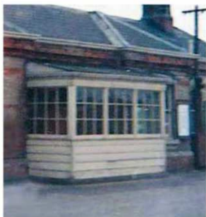
This slightly damaged picture shows the storm porch which apparently dated from the 1930s and lasted until the 1960s modernisation. CHRIS LEIGH
