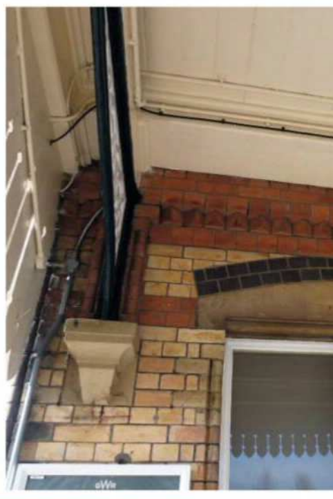
Detail view of the window, lintel, decorative brickwork and under-side of the canopy.
