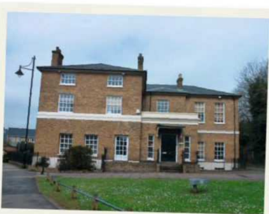
Now: The front of the former station as it is today. It would now yield little to assist in building an accurate model of the station as it was. In addition to the obvious changes, the window style has been changed, the rendering and small porch removed and a basement level added. CHRIS LEIGH
