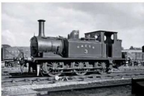
KESR No. 3 Bodiam at Rolvenden on September 24 1947. The locomotive sports a unique bunker, fitted in 1932. It was also fitted with an 'A1X' boiler at the KESR's own workshops, with help from the Southern Railway. J.M. JARVIS/ONLINE TRANSPORT ARCHIVE/RAS
