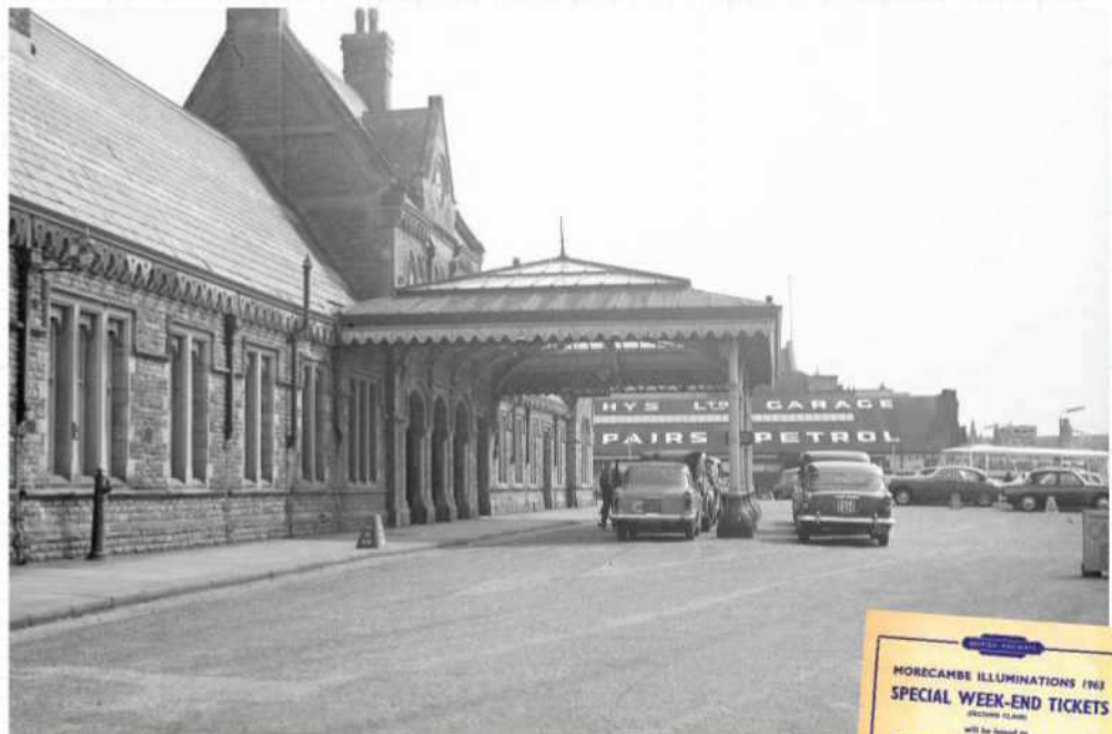
Promenade station was built from sandstone with a blue slate roof and has a partly glazed canopy with a pitched roof on four cast iron columns. Photographed on June 5 1965, it closed in 1994 and was replaced by a new station closer to the town. This handsome structure still survives.
