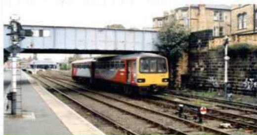
Belgrave Terrace Bridge and the accompanying shallow cutting, with its impressive stone retaining wall, are an essential feature. The beautiful sand-coloured housing, on the far side of Westwood (road), was reluctantly omitted to provide a clear view of the line.
