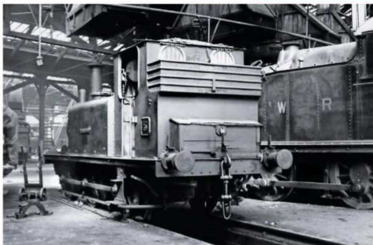
Could William Stroudley ever have foreseen this? Western Region 'A1X' No. 5 Portishead rests in the roundhouse at Bristol St Phillips Marsh alongside a '56XX' 0-6-2T, on March 29 1948. RAIL ARCHIVE STEPHENSON
