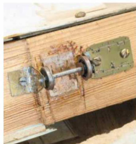
A set of brass W-irons and a set of wheels is secured to the bottom of the sector plate, supporting the track as the plate pivots on its fixed axis.
