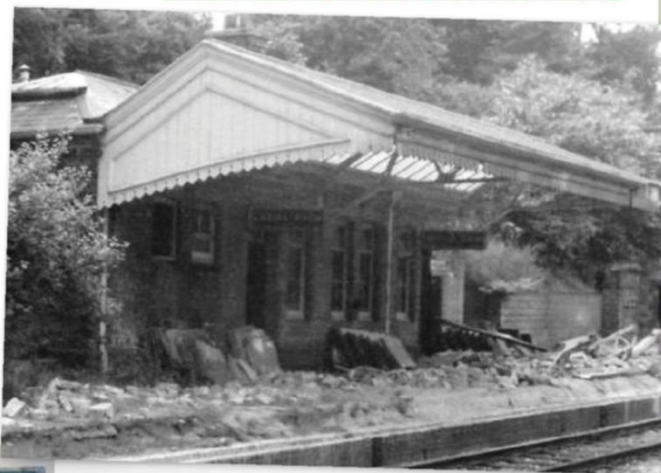
Above: The Down side building at Savernake Low Level was similar to the structures at Lavington. It comprised two waiting rooms, the Ladies Room being separate. CHRIS LEIGH
