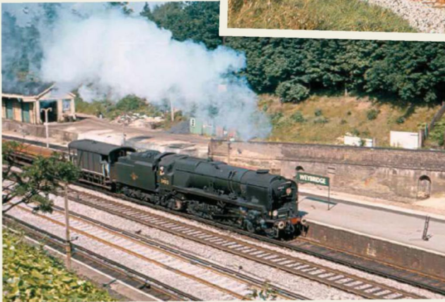
Rebuilt 'West Country' 4-6-2 No. 34013 (formerly Okehampton) heads a long-welded rail train on the Up Slow at Weybridge during the Bournemouth electrification works. The Down Fast has been relaid with concrete sleepers and both Fast lines have fresh ballast, though not the Slow lines. KEITH JAGGERS
