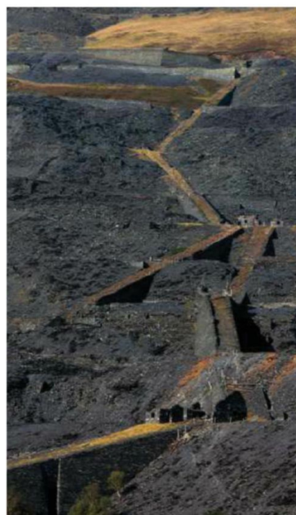
One of the disused inclines in the former Dinorwic quarry at Llanberis, built on slate embankments. The inclines linked the different working levels, called galleries. ATGOF.CO/ALAMY
