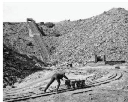
A view of one of Pen-yr-Orsedd quarry's inclines, photographed on October 20 1968, with the winding house at the top. Of interest here is the mixed gauge track; within the quarry a nominal 2ft gauge was used, while the connection to the outside world was via the 3ft 6in gauge Nantlle Railway. KEITH JAGGERS
