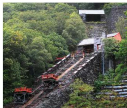
The National Slate Museum, at the former Dinorwic Quarry, has a short section of restored incline. Wagons are carried side by side on a lifting table, rather than cables being attached to 'runs' of wagons. DOMINIC JONES/ALAMY
