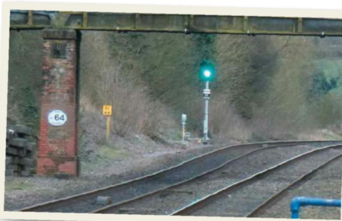
A four-aspect colour light signal on the Up line at Kings Sutton on the approach to Aynho Junction. CHRIS LEIGH
