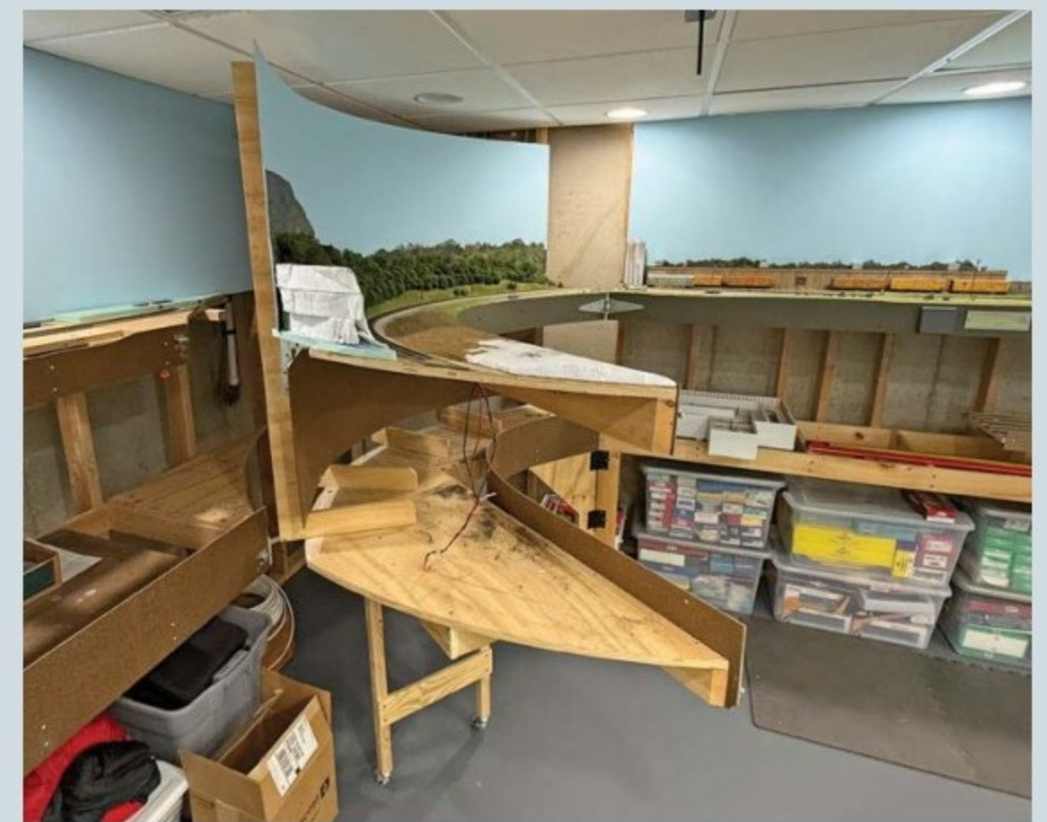
A swing gate, based on a similar design Tony Koester built for his NKP layout, provides easy access to the home's electrical panels.
