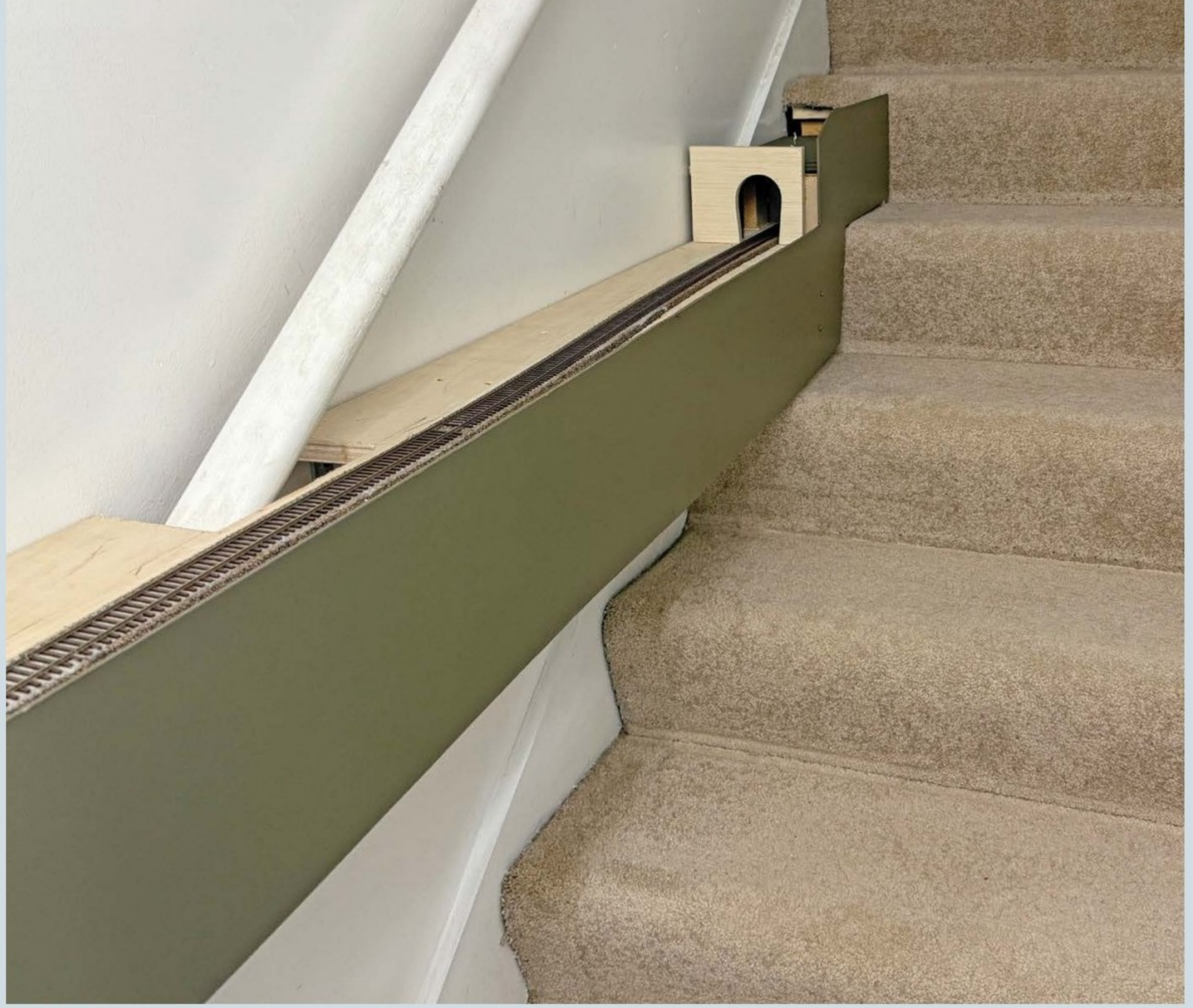
The main line navigates the stairs via a tunnel that was cut through the staircase. This allows unencumbered entry into the layout room.
