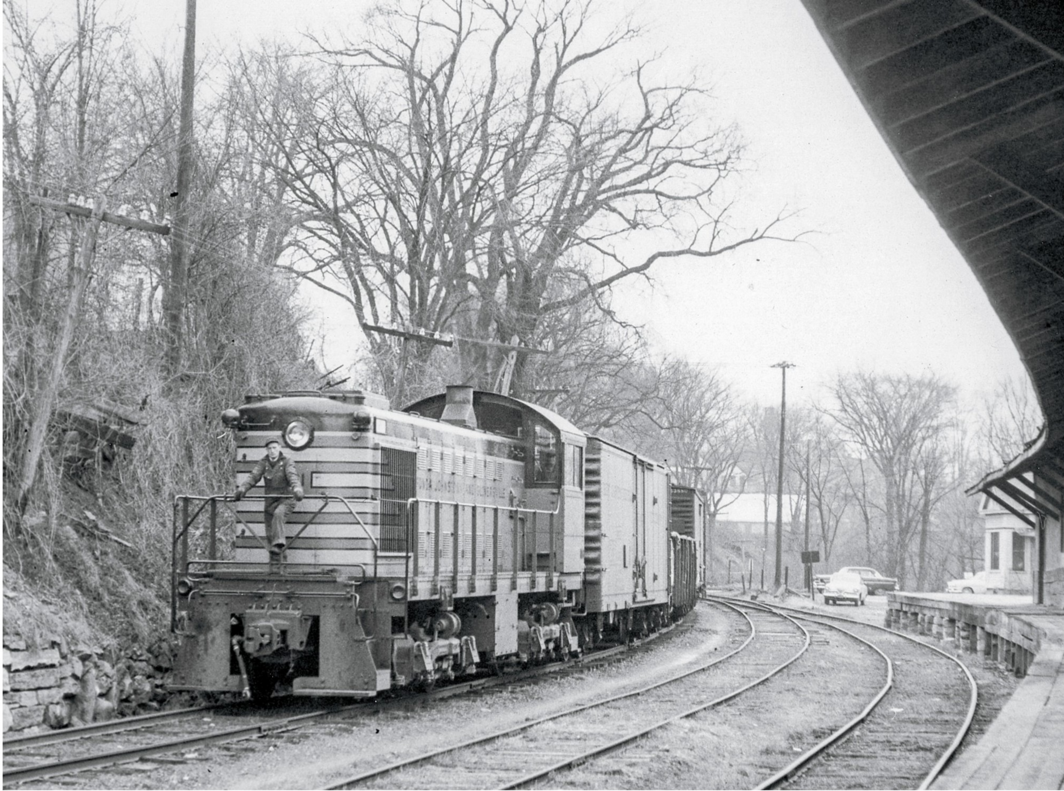
A Fonda, Johnstown & Gloversville train rumbles past the freight house in Johnstown, N.Y. Paul Boehlert designed an HO scale track plan based on the shortline railroad. Photograph by Jim Shaughnessy, collection of the Center for Railroad Photography & Art, www.railphoto-art.org
