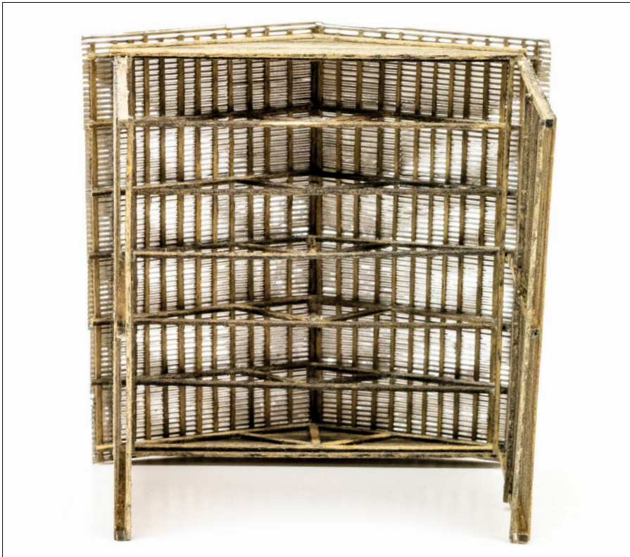
This inside view of the roof shows how it's supported by 2 x 4 trusses. A jig would simplify building the trusses.
