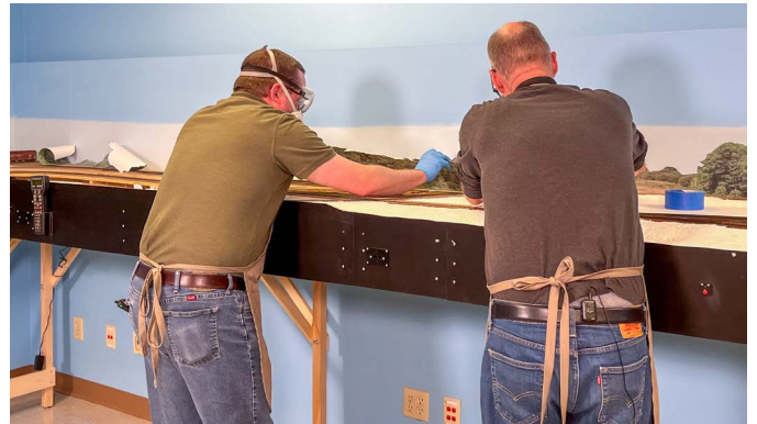
It takes two people to position and apply long sections of backdrop because the adhesive will stick as soon as it comes in contact with the painted hardboard.
