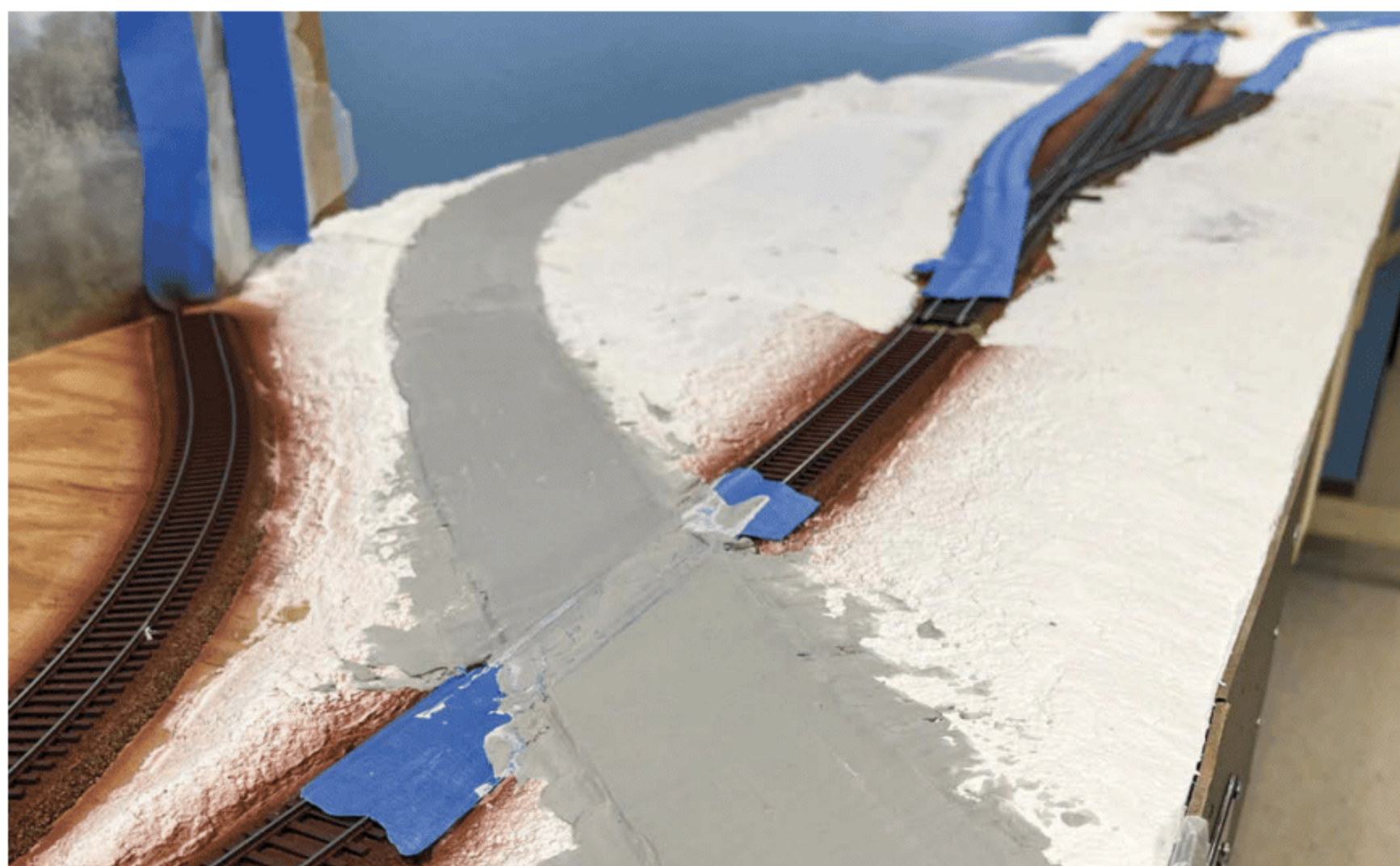
The road's surface is made with Woodland Scenics' Smooth-It plaster tinted with Earth Colors Slate Gray acrylic pigment.
