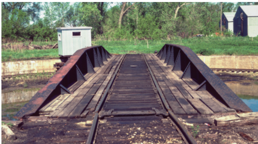
Taken in 1984, this photo shows the replacement cab for the tractor. Note the stained and weathered walkway boards and the rail lock spanning the track gauge at the end of the bridge.
