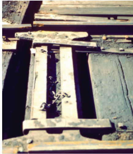
The rail lock mechanism helped hold the turntable in alignment with the radial tracks around the pit.
