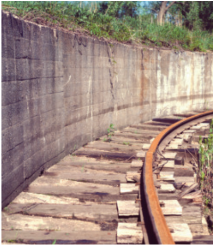
The detail of the pit wall shows the impressions of the wood forms used to pour the concrete.
