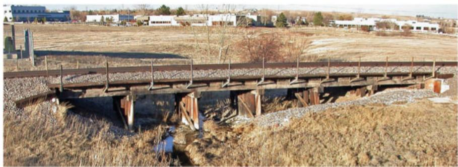
① The prototype pile trestle has a ballasted deck and a walkway with a steel cable railing on one side as shown in this early spring view.
