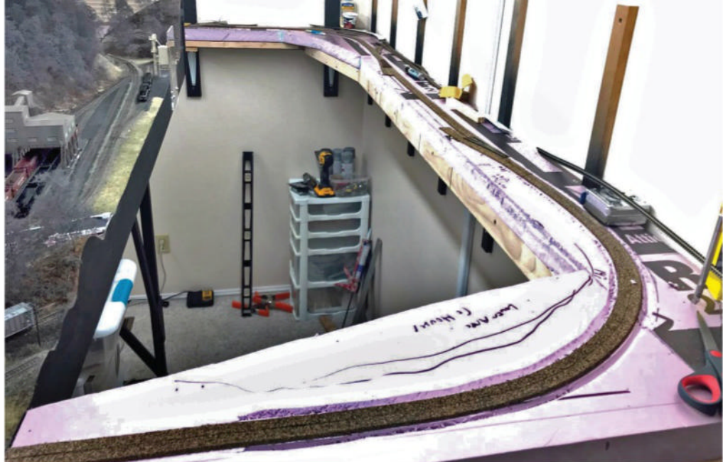
11 Part of the Slate Fork Branch's right-of-way comprises a narrow shelf built from foam-covered hollow-core doors mounted on shelf brackets. The brackets are attached to 1 x 2s that also support the hardboard backdrop.
