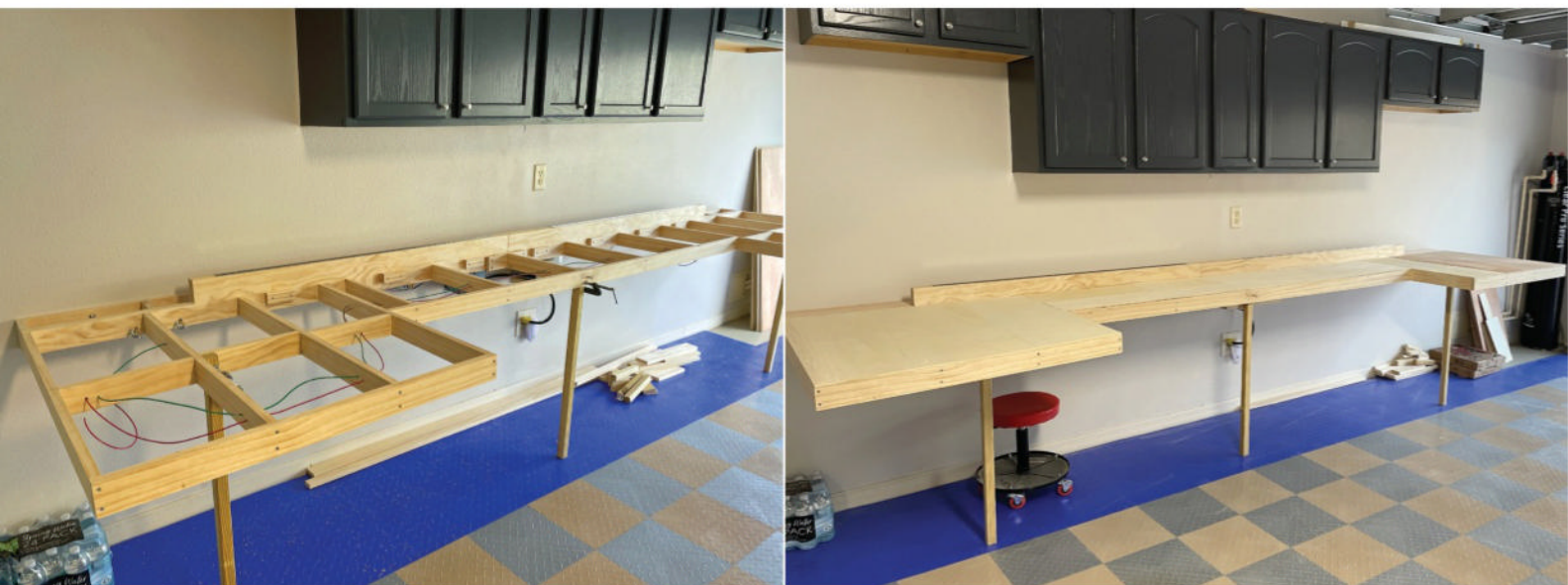
Two views of the benchwork under construction show the sturdy framing and the two long piano hinges running along the raised “backbone.” Note the notch in the benchwork to fit around the wall cabinets. The removable legs fit into sockets.
