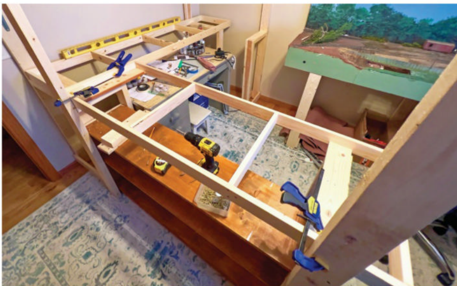
The benchwork for the stacked two-deck layout was designed to be completely self-standing. In this early construction photo, Joseph has built the support legs from 2 x 4s and the benchwork framing from 1 x 4 pine boards. The upper deck is supported by heavy-duty shelf brackets. A section of his previous On30 layout is already in place.
