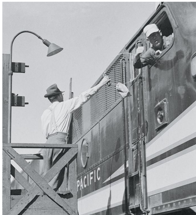
Atop what Northern Pacific railroaders called "the pulpit," the Stampede operator passes a staff as if hooping up an order in July 1945. The pouch dangling from the hoop contains the staff. J. M. Frederickson photo, courtesy of Pacific Northwest Railroad Archive, JMF02-03725
