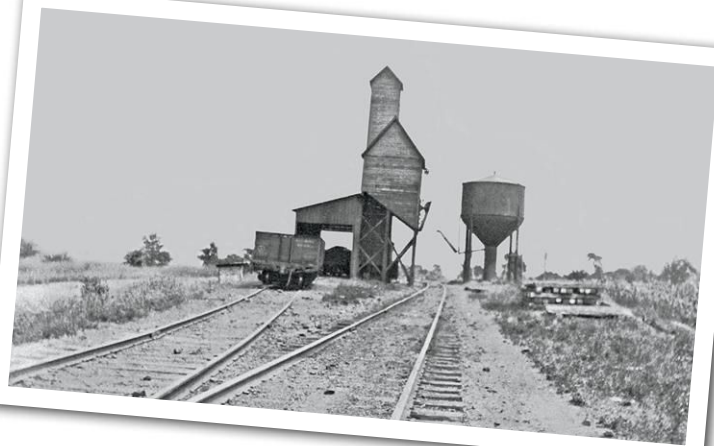
This vintage photo of the Nickel Plate's Cayuga, Ind., water tank and coal dock shows just enough detail to indicate the spout was supported by bracing between two of the tank's four legs. The pipe to the spout angles downward. Clyde Eyrse collection courtesy Steven Grigg
