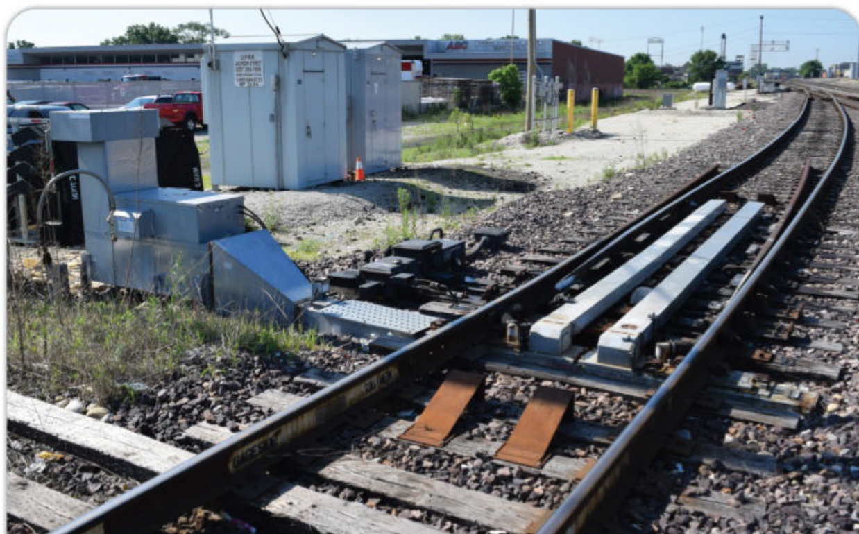
A hot-air-type switch heater protects this switch-style derail from freezing up in winter. The combustion chamber, stack, and air handler are at left. Ducts in the gauge of the track route hot air against the side of the rails. M.R. Snell photo
