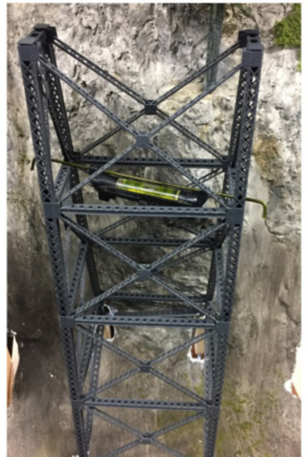
13 Here, the new bridge is being installed. Building the towers off site and only installing one tower and span at a time assured only brief operation outages occurred.
