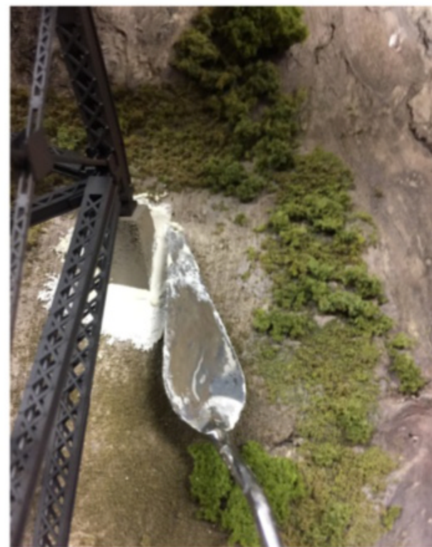
16 After the first revenue trains successfully crossed the bridge without any issues, new hardshell was troweled in place between the existing hard shell and the tower plinths, finishing the installation.
