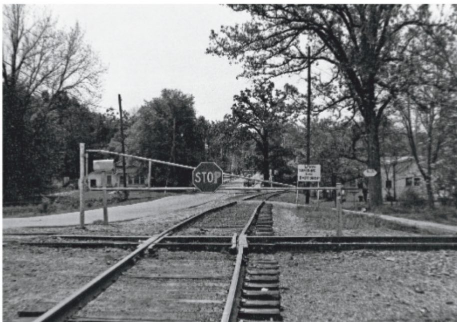
① Prototype example. A pipe gate with a stop sign attached protects the junction of the Ashley, Drew & Northern and Missouri Pacific in Monticello, Ark. The gate is lined against the AD&N. Terry A Holley photo
