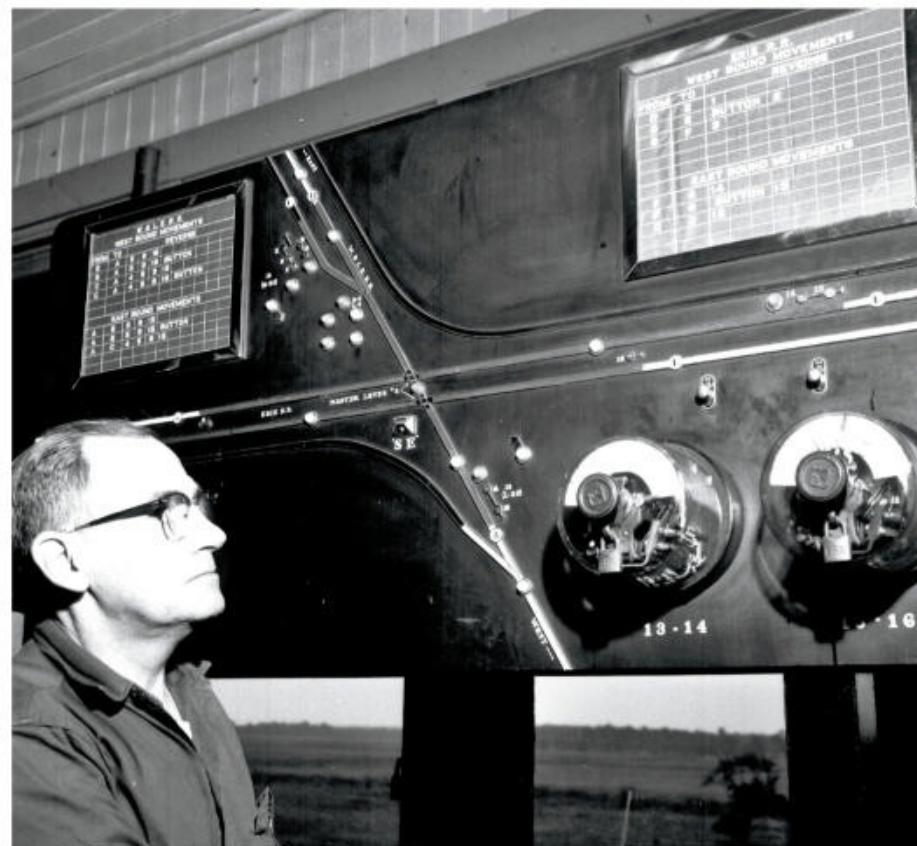
Operator Vernon Caston watches the model board at SE Tower in Creston, Oh. in June 1957. SE guarded Wheeling & Lake Erie's crossing of the Erie there. John Long photo from the Dan Biernacki collection
