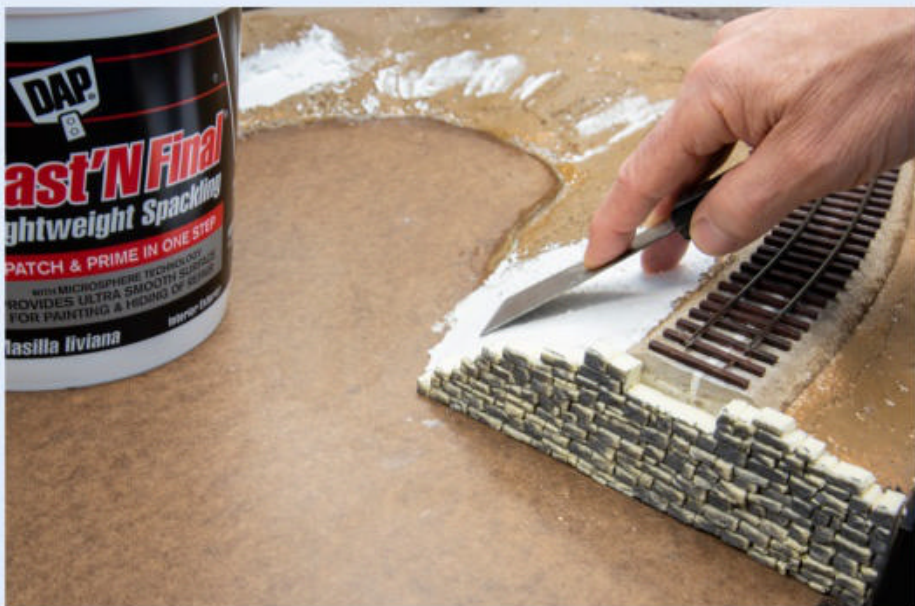
9 After putting the bridge abutments in place, Lou backfilled them with lightweight spackle.
