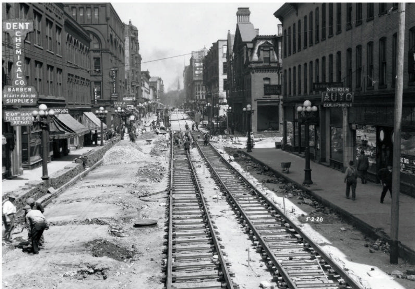
On May 2, 1928, crews were busy rebuilding a section of trolley track in downtown Grand Rapids, Mich. Modeling such a scene offers myriad detailing opportunities. Photo courtesy Grand Rapids, Mich., City Archives and Records Center
