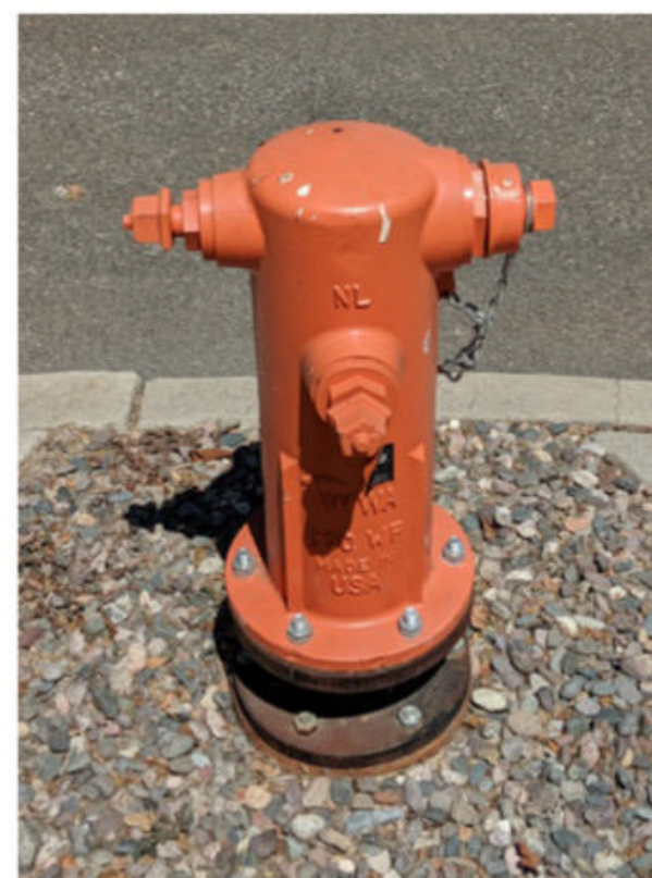
4 Wet-barrel hydrant. Water is present in this style of fireplug, which is used in warmer climates.
