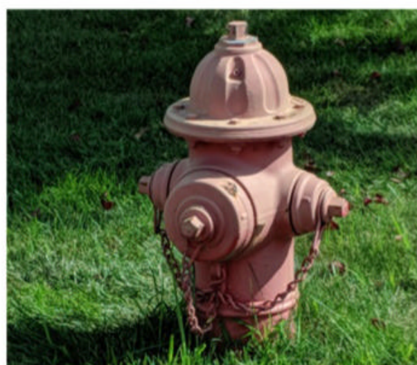
5 Dry-barrel hydrant. This style of fireplug is common in colder areas. The valve nut on the hydrant's top connects with a valve buried in the street.
