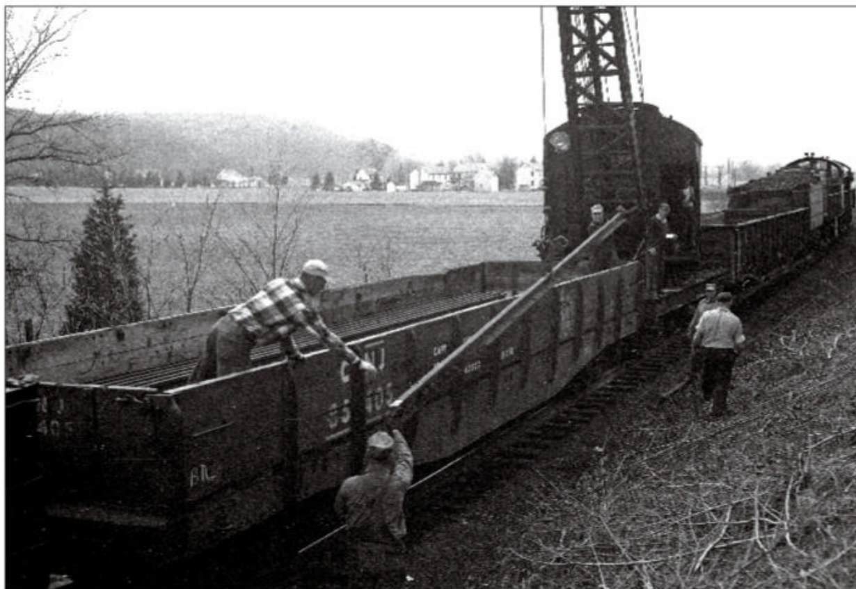
John Treen, a veteran New York Susquehanna & Western conductor, captured many "insider" views of railroading. On April 9, 1951, two section foremen and their men are loading scrap rail with Work Extra 252 at Vails, N.J. John L. Treen photo
