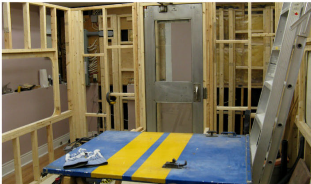
The side doors required extensive refurbishment and copious amounts of body filler. The end door is so heavy that the jambs had to be anchored to the ceiling joists for stability.
