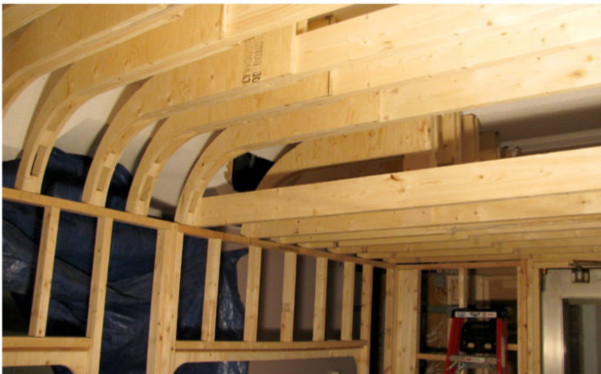
Pieces of plywood cut to the interior and exterior profiles were laminated to 2 x 6 lumber to form the ceiling. Jason would have used 2 x 4s if he were doing it again.
