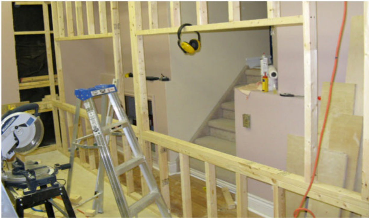
The coach was framed with inexpensive 2 x 3 SPF (spruce/pine/fir) lumber. Jason laid the plywood floor directly on top of the existing laminate flooring.
