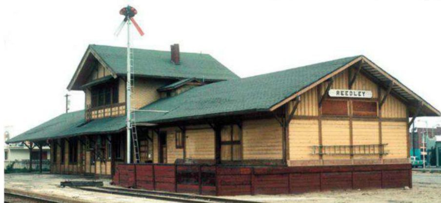
The Southern Pacific's Reedley depot had a green shingle roof that adds a nice bit of color to the building. An elevated freight platform is built around this end and along the track side. Here, too, there's a bay window in the operator's office and a lower-quadrant train order signal. John Signor photo
