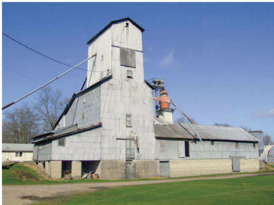
The Wolcottville elevator is along the former Pennsylvania RR’s Grand Rapids & Indiana line. According to the elevator operator, the elevator in this April 2007 photo looked pretty much the same in the mid-1950s, the era Jim models.
