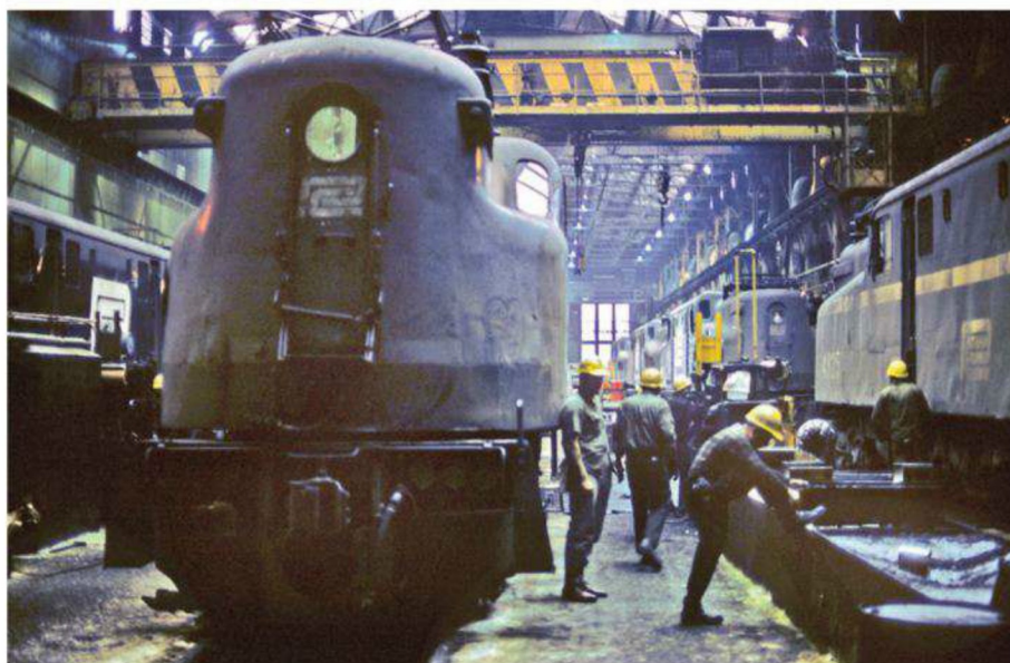
A gritty interior added a lot of atmosphere to the GG1 electric locomotive shop in Wilmington, Del., in 1972. The aisle could be in the foreground.
