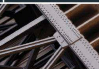
72' Deck Plate Girder Bridge
