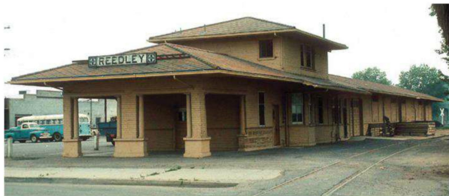
Santa Fe’s Reedley, Calif., depot was a large structure. Looking down the platform we can see the angled operator’s bay, an elevated trackside freight platform, and a large freight-house addition at the far end. John Signor photo
