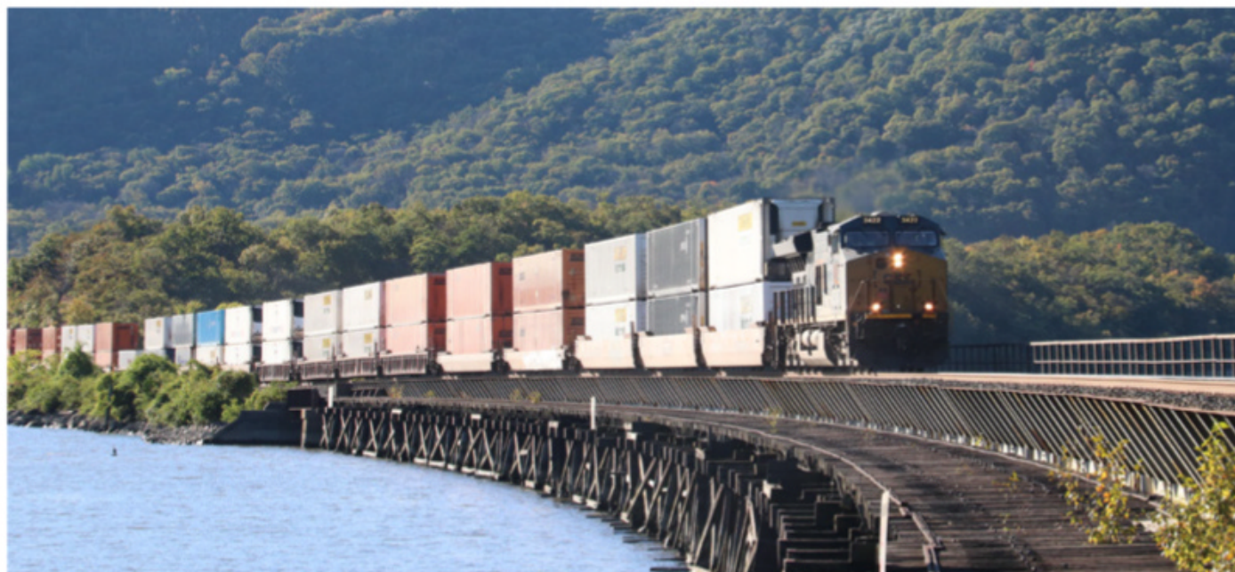
CSX’s scenic River Subdivision along New York’s Hudson River is Centralized Traffic Control territory, so signal indication authorizes movements like this northbound freight crossing the Iona Island trestle on October 18, 2018. Jerry Dziedzic photo
