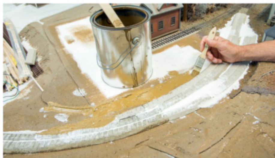
5 Earthworks. Lou laid new 1/4" Homabed under the main line and 1/8" Homabed under the sidings. He filled voids with spackle, then added a coat of earth-tone latex paint.
