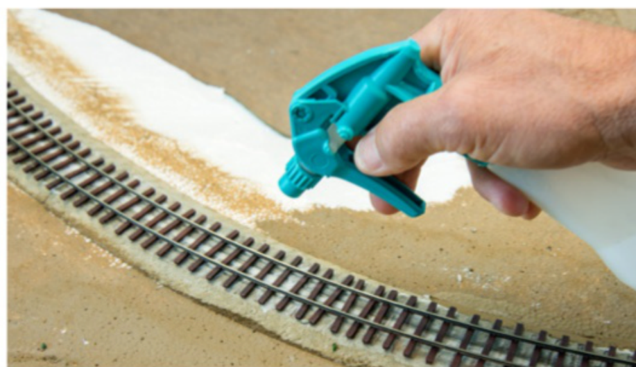
3 Water-soluble to the rescue. Spraying everything with water allowed Lou to loosen the track, which was held down with white glue.
