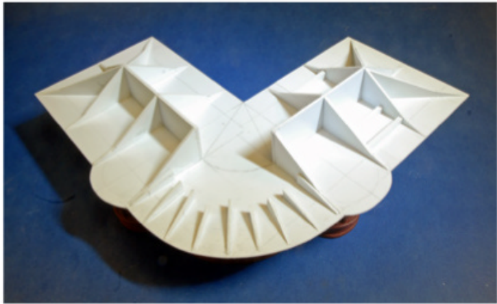
4 The station roof is a cranked or compound hip, which means the corner is two overlapping quarter cones.
