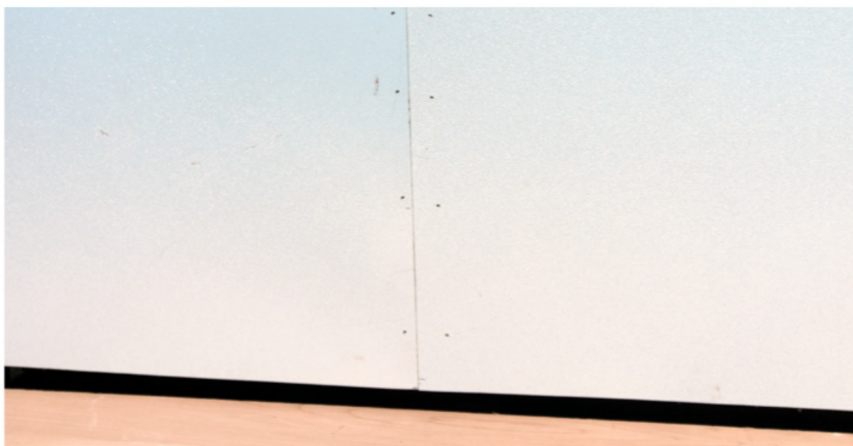
Fig. 3 Mounting the hardboard. The ends of the painted hardboard backdrop sections are butted together and fastened to 2" x 2" joists with nails.
