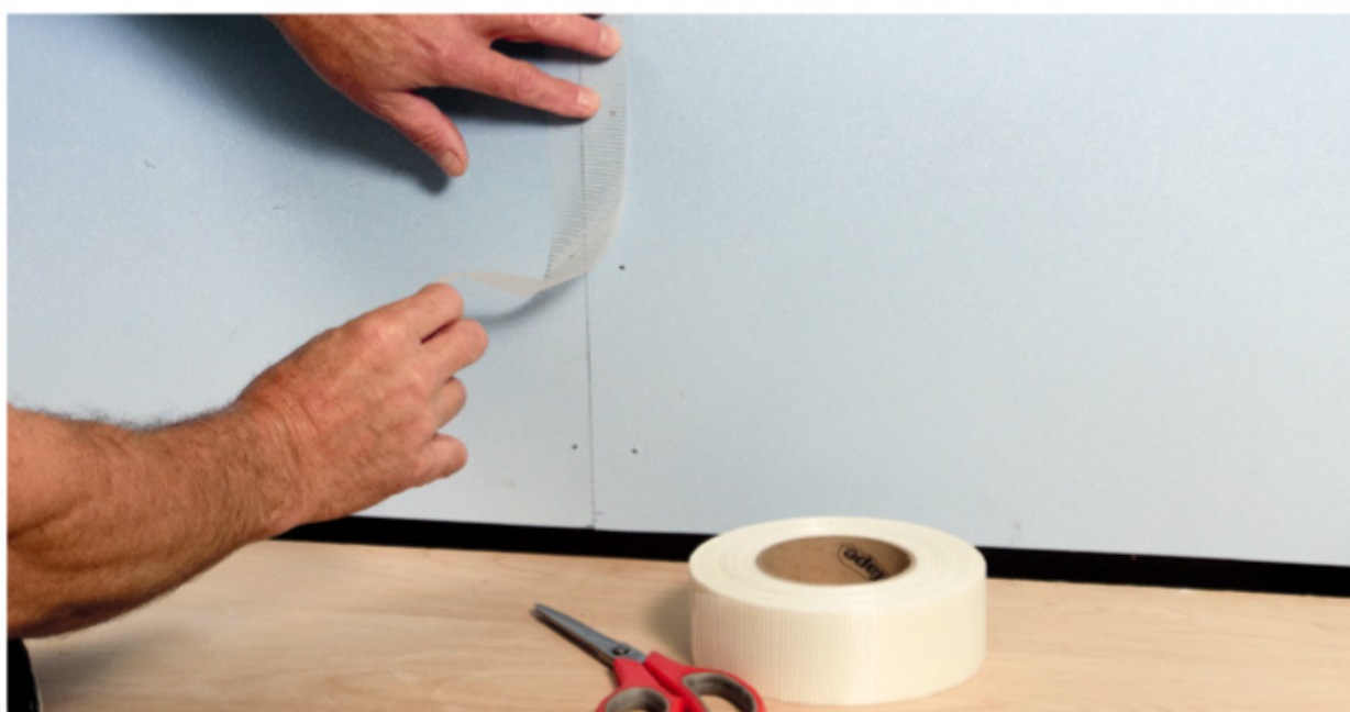
Fig. 4 Taping the seam. Gerry applies self-adhesive Fiberglas mesh tape over the gap between backdrop sections and nail holes. Paper tape can also be used.
