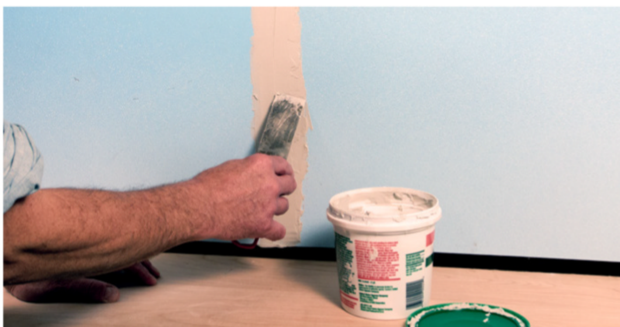
Fig. 5 Mudding. Wallboard joint compound ("mud") is applied over the mesh tape and feathered about 1/2" on either side. Don't worry if it's not smooth.
