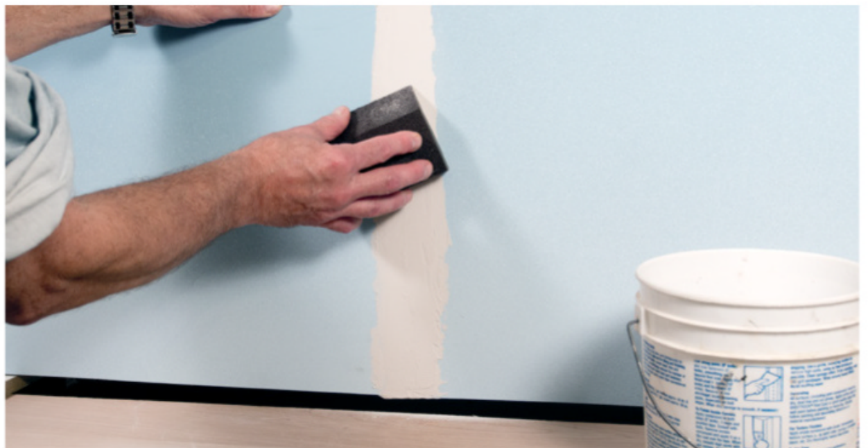
Fig. 6 Sanding it smooth. When dry, the mud is sanded, hiding the seam and nail holes. Mud may need to be re-applied and sanded for a good finish.
