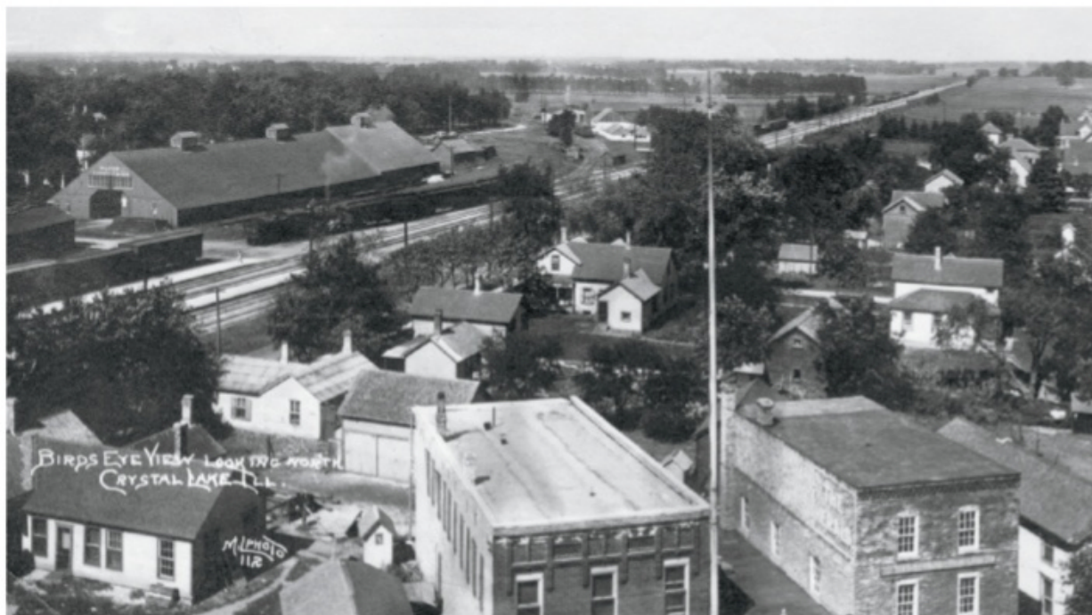
This undated view of the enclosed lumberyard was taken from atop the city's wood water tower sometime in the early 1900s, before the new depot was built. The massive lumber shed was about 90 years old when it was taken down in the 1980s. Photo provided by Diane Kenney, Crystal Lake Historical Society
