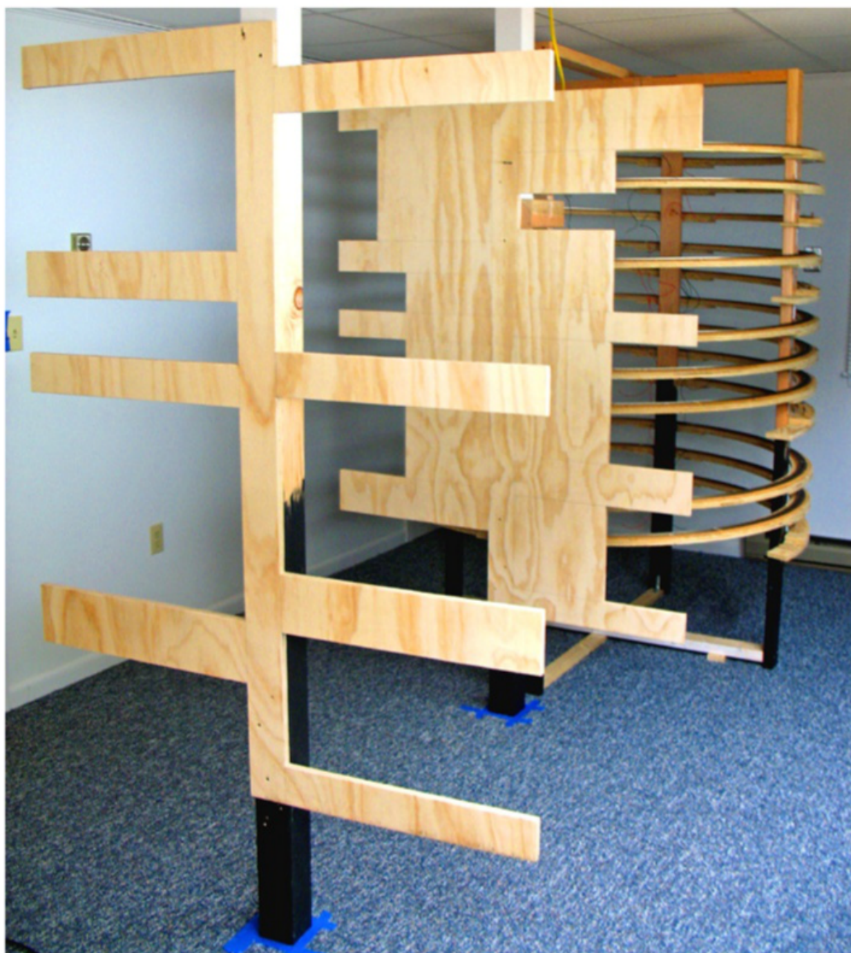
6 Joe wanted easy-to-build and strong brackets to support the numerous decks of a peninsula required by the expanding design, so he cut them from \frac{3}{4} " plywood. He mounted them to 4 x 4 posts secured to the floor joist above by slip joints to allow for movement of the layout as humidity changes.
