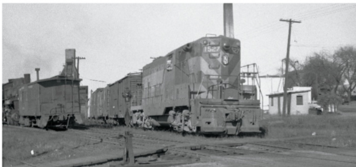
This 1953 photo shows the local switcher and caboose on the grade that runs up to the depot as C&NW GP7 no. 1527 leads its train along the Geneva Division. The smokestack and buildings behind the Geep belong to the Bowman Dairy. Eugene Lewis photo, courtesy of the Chicago & North Western Historical Society
