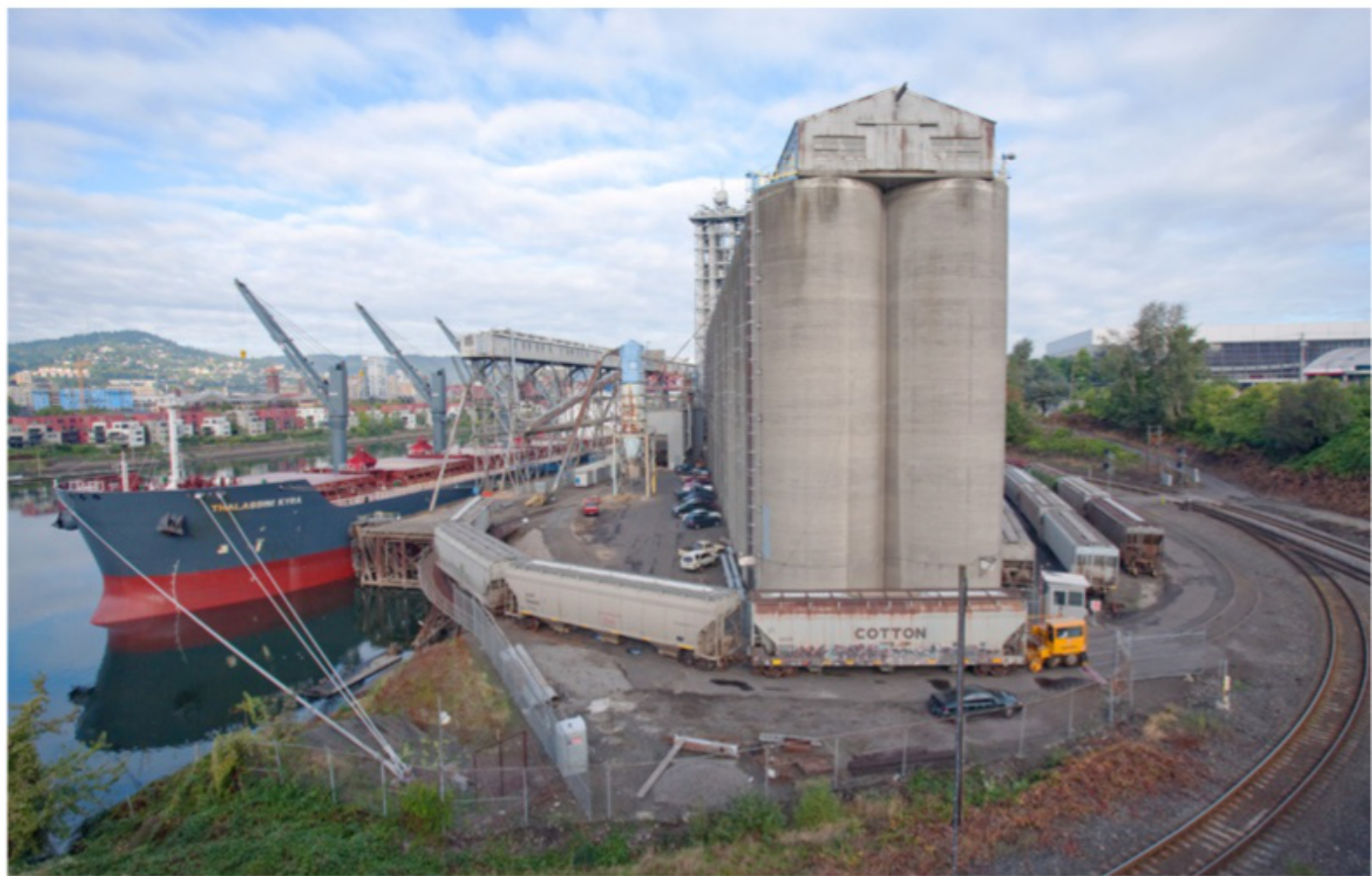
What looks like a curve found only on a model railroad is found at CLD Pacific Grain's dock on the Willamette River in Portland, Ore. A Trackmobile is pulling four covered hoppers around the loop track. The track in the foreground connects to the Steel Bridge over the Willamette River. Scott Lothes photo
