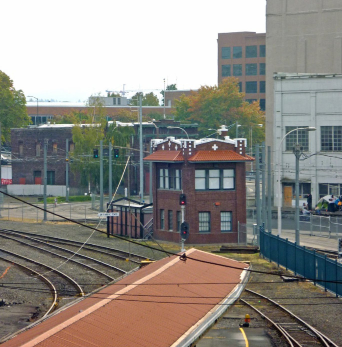
The interlocking tower at the eastern end of Portland Union Station is ornamented in the same architectural style as the main buildings. Iain Rice photo
