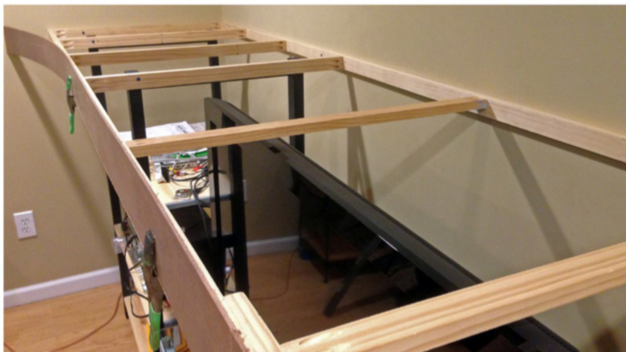
Ikea's Ivar shelving forms lightweight, but sturdy, benchwork when attached to the wall. The shelving below the layout is an added bonus.
