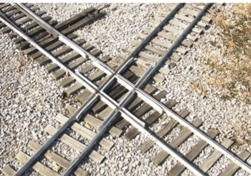
Outdoor railroading at 7½" gauge needs some big track. The Grossers build their track in panels using 1" aluminum rail screwed to 16" ground contact treated wood ties.
