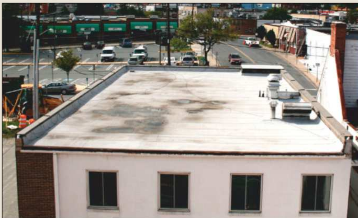
Judging by the gray color, this is probably a single-ply membrane roof surface.
