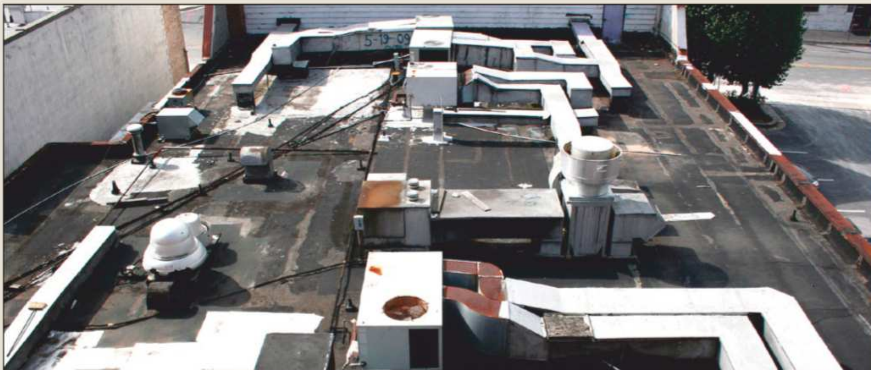
The black color and seam pattern suggest that tar paper rolls cover the roof.
