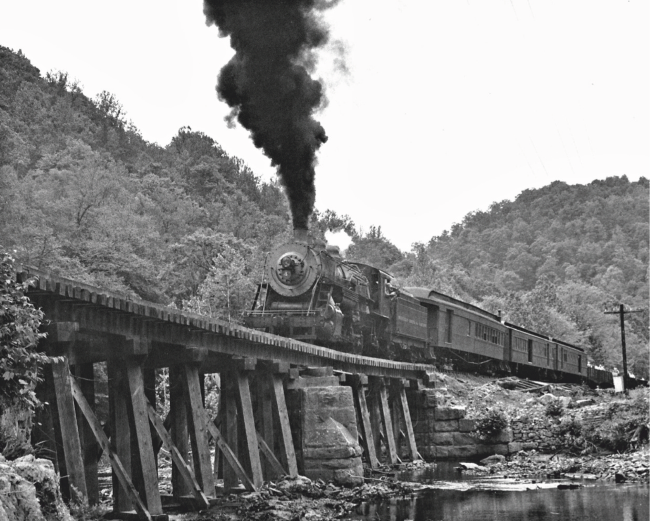
The Sand Fork bridge, with its temporary timber bents, supports Buffalo Creek & Gauley no. 4 as it pulls a National Railway Historical Society fan trip extra in 1955. Doug Andre photo
