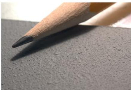
❸ The pencil in this enlarged photo of a wall section demonstrates how fine the spray adhesive texture really is.
