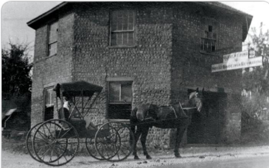
The walls of the prototype building, which is constructed of fieldstone cobble, are a hefty 24 inches thick. Photo courtesy Richard Palmer
