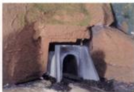
Fig. 5 TUNNEL PORTALS. The south portal (prototype and model shown above, top row) is concrete with stone block retaining walls, while the north portal (prototype and model bottom row) has a stone face with poured concrete retaining walls.
