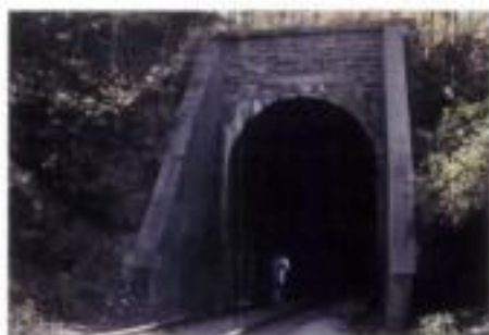
Fig. 5 TUNNEL PORTALS. The south portal (prototype and model shown above, top row) is concrete with stone block retaining walls, while the north portal (prototype and model bottom row) has a stone face with poured concrete retaining walls.
