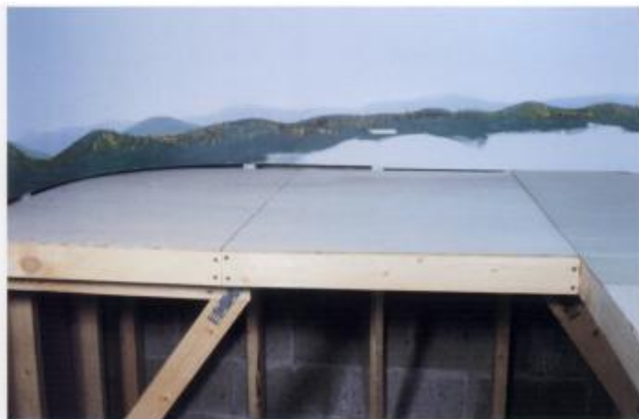
Fig. 5 TABLETOP. The tabletop sections are simply 1 x 3 frames with \frac{1}{8} " plywood tops. Use drywall screws to hold them together.
