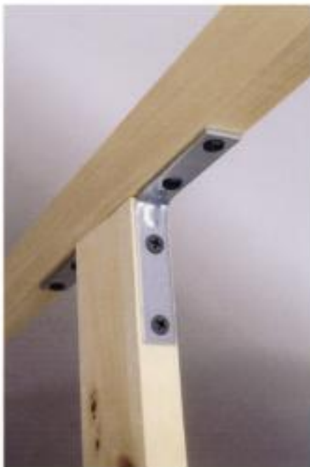
Metal L brackets help to keep the backdrop frame rigid. These are held in place with drywall screws.
