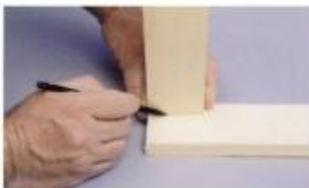
Lionel notched the backdrop support in a couple of places. Here he's using a scrap piece of 1 x 3 to trace cut lines on the support. He then cut it out with a jigsaw.
