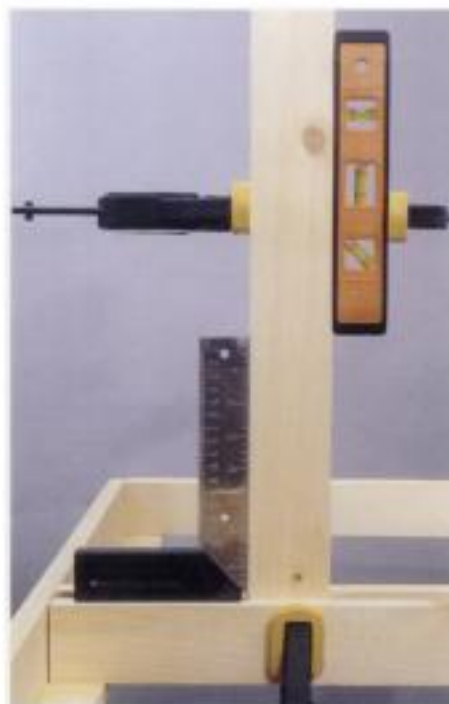
The backdrops are supported by 1 x 3s run perpendicular to the benchwork.
