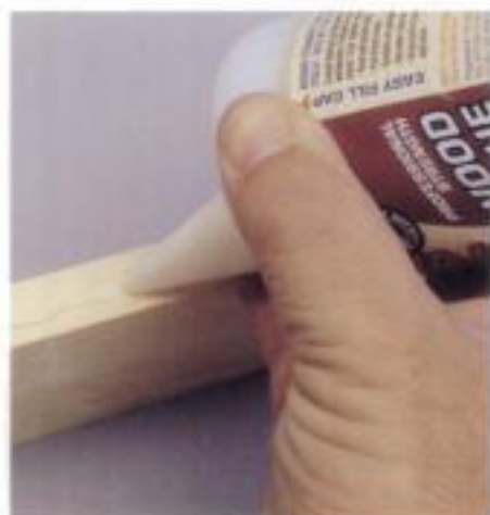
Whenever possible add a thin bead of carpenter's glue to provide added strength to the frame.
