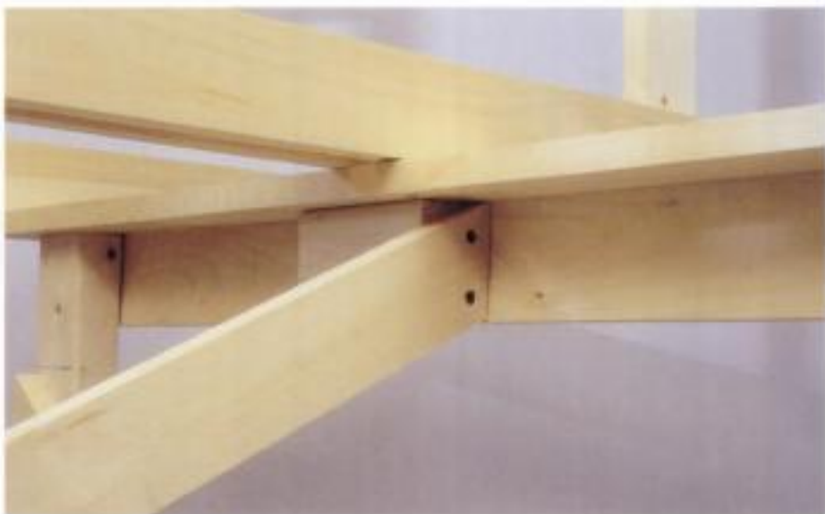
Drywall screws, installed using a cordless screwdriver, make benchwork assembly go very quickly.
