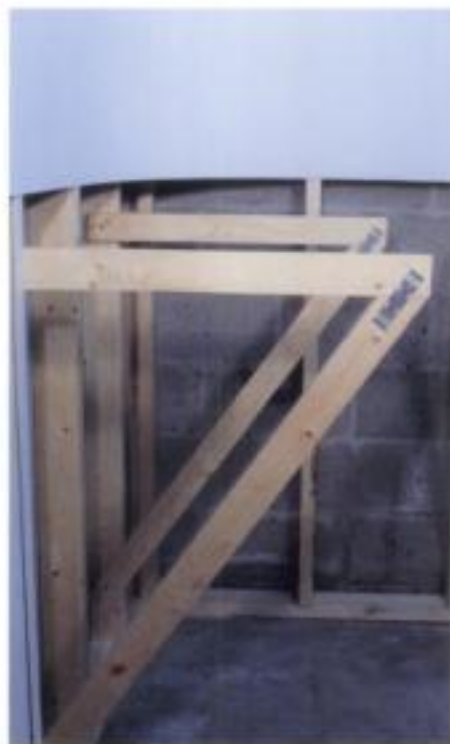
Fig. 4 BRACE. The angled braces are made from 1 x 3s as shown in the drawing above. Be sure the tops are level when installing them.
