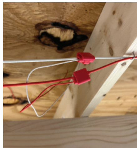
Under the layout, the feeders are attached to the 16AWG bus line using insulation displacement connectors.
