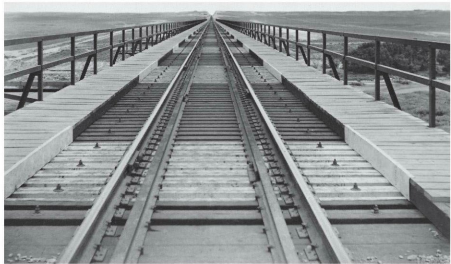
Fig. 3, above. This open floor system on a deck truss bridge over the Cimarron River in Kansas was built in 1938 by the Rock Island. The walkway planks running the length of the structure are covered with an additional crosswise layer. Guardrails placed inside the running rails help to keep derailed wheels in line. Fig. 5, below. A through plate girder bridge with a ballasted floor built by the Baltimore & Ohio RR to eliminate a crossing over a highway. Ballasted flooring provides a smoother roadbed than open flooring.
