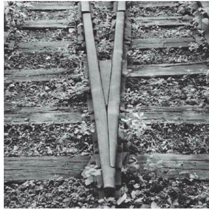
Fig. 6. Guardrail ends are terminated in several ways. Looking from left to right, the rail ends are brought together and bent down into the ballast,
