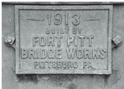
Fig. 14. An example of a bridge builder's plate. These are cast-metal plates attached to an end of the bridge structure. Plates on large bridges may give information about the location and the designers and politicians involved in the project.
