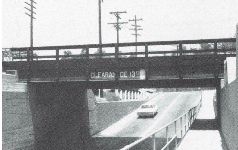
The west side of the bridge has a plain 24" I beam showing instead of the concrete facade. Since this view was taken in 1972, Santa Fe maintenance forces have painted the girder light blue to make it more visible to drivers.
