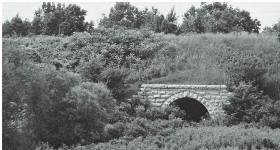
Fig. 5. Stone arch culverts are essentially identical to concrete ones, but the wing design differs. Stone culverts have stepped tops, while concrete ones have straight wings, as seen in fig. 4.
