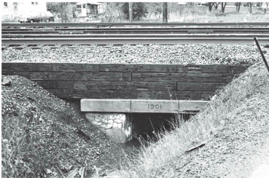
Fig. 3. A simple rectangular culvert made of concrete slabs, with timber sidewalls to retain the ballast.
