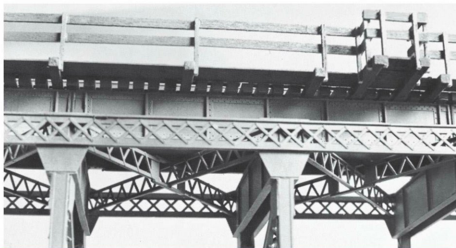
Construction of fascia and cross-bracing lattice
