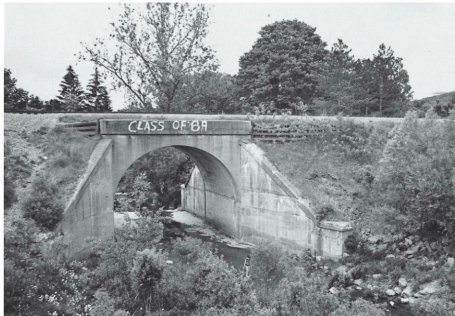
Fig. 4. Like most arch culverts, this concrete structure on the Nickel Plate Road has an opening designed to handle high water. Tapered wings are applied to both ends to control the flow of water.
