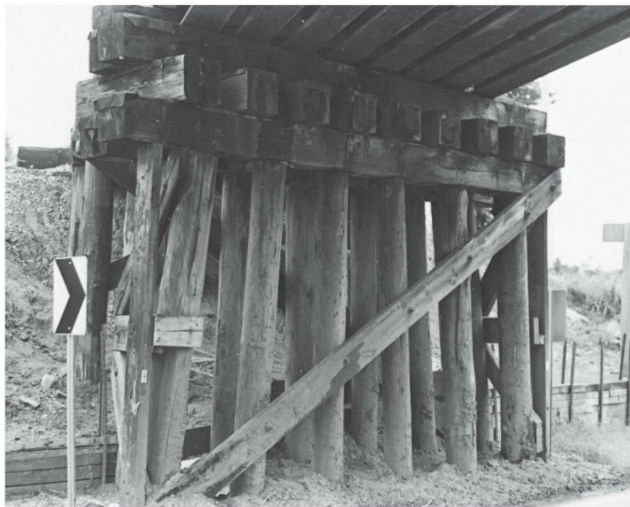
Fig. 5. Timber trestle bents are sometimes used to support steel bridges, as in the case of this Toledo, Peoria & Western RR bridge near Le Harpe, Ill. To distribute the load between there are short crosswise timbers between the bent caps and the single cap supporting the steel beams of the floor.
