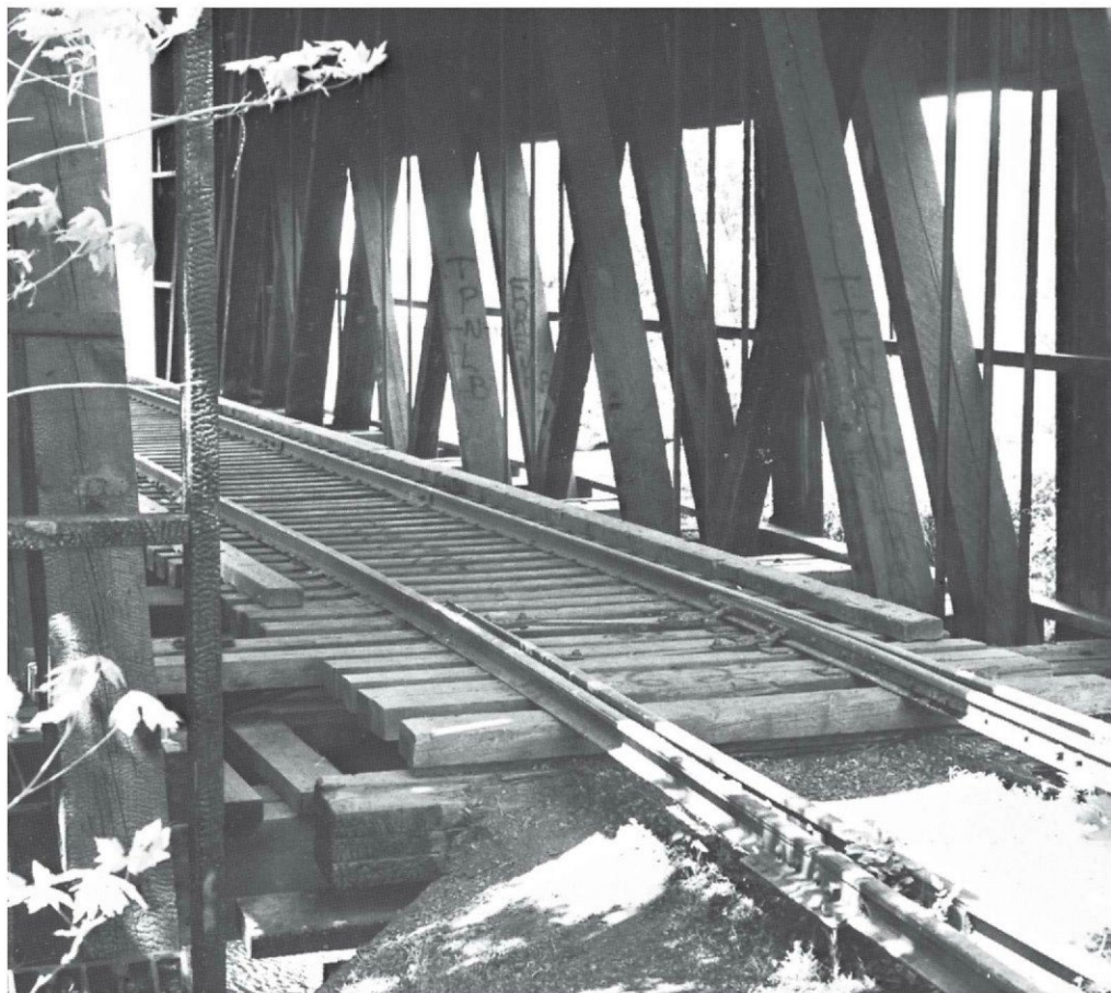
The unusual switchpoints on the east end of the bridge are explained in the text. Notice the graffiti: "TP-n-LB Forever" and "Tina-n-Lars." Note, too, in the left foreground, that this end of the bridge has been burned, but apparently it was a minor fire that was quickly extinguished. This view also shows the spacing of the vertical truss rods, grouped in threes.
