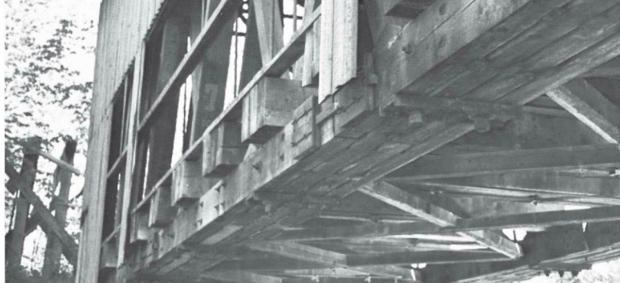
This photo clearly shows how the beam tension fittings were built and also shows the mortising of the crosspieces. The bolted channels are the vertical truss rod tension fittings.
