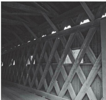
Fig. 13. A vertical plank wall covers the interior lattice trusses of this covered highway bridge. Windows were sometimes cut into the sidewalls.
