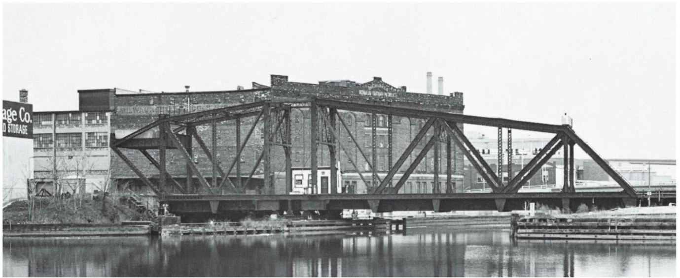
Fig. 11. Built in 1904 for the Milwaukee Road, this offset center-bearing swing bridge over the Menomonee River in Milwaukee, Wisconsin, has a heavy concrete counterweight at the left to keep the bridge in balance.
