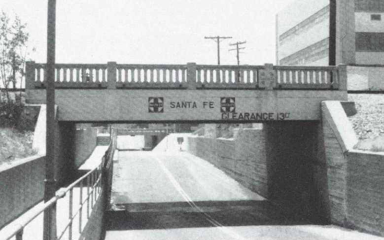
This view of the east side of the original bridge, photographed in 1972, includes a square sheet metal Santa Fe emblem on the railing. This sign was bolted in place with wood blocks serving as spacers around the cast post.
