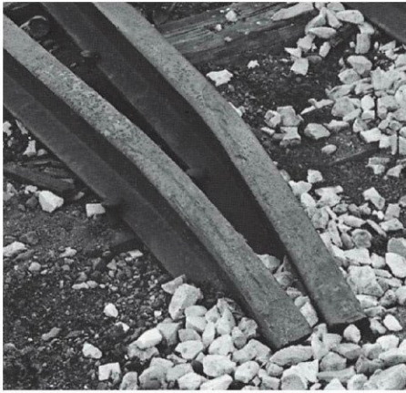
Fig. 6. Guardrail ends are terminated in several ways. Looking from left to right, the rail ends are brought together and bent down into the ballast,
