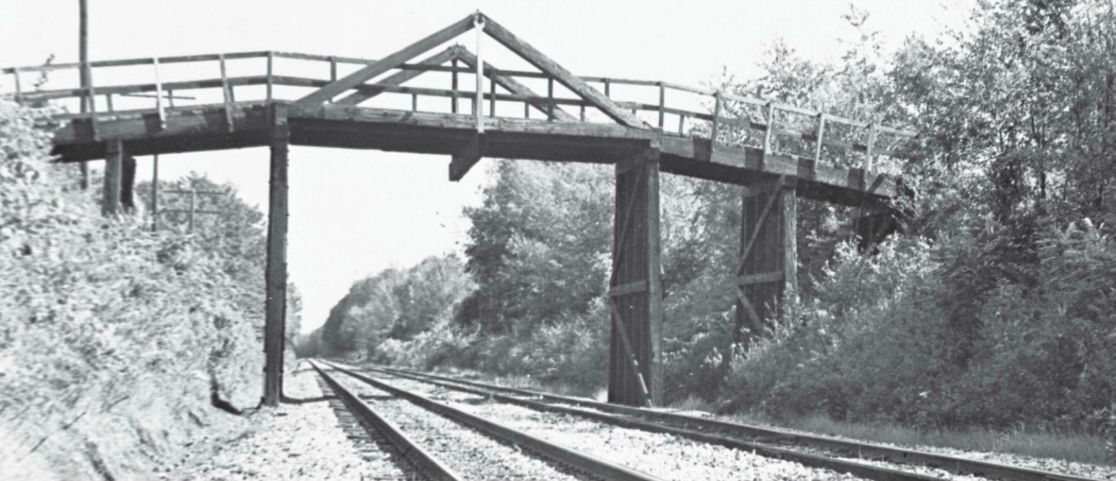
This quaint old wooden king-post truss bridge spans a double-track section of Conrail (old Nickel Plate Road) trackage in western New York State. Harold Russell photos
