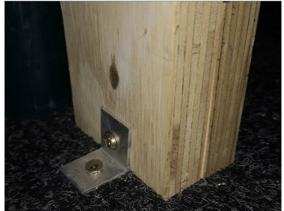
5. Securing to the floor.
